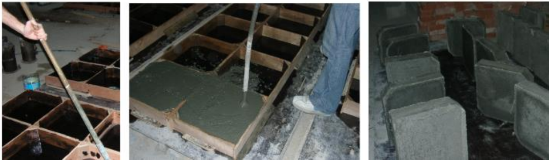
Figure 5.3-2: Test Specimens. Reprinted from ‘Retrofit of concrete panels with prefabricated HPFRCC plates’ by I. Bedirhanoglu, A. Ilki, O. Incecik, N. Kumbasar , 2008.
