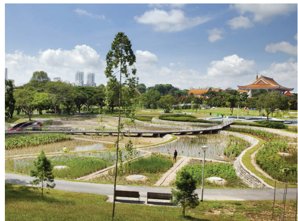
Figure 6.23: Biofiltration Terraces at Bishan Ang Mo Kio Park. These biofiltration terraces create extra space for flood waters to fill (Ramboll Studio N.D.).
