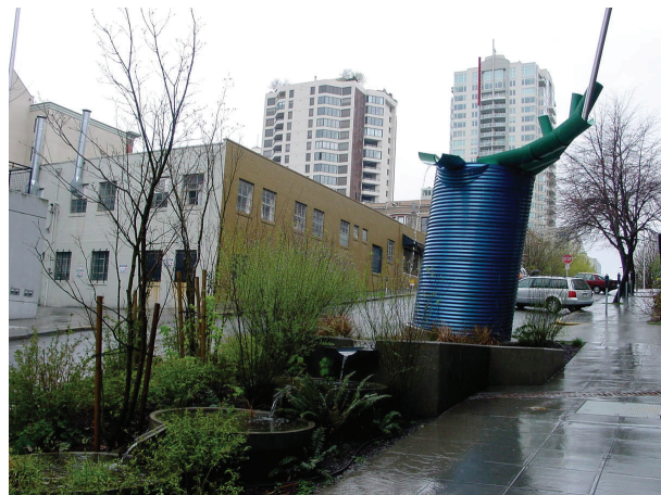
Figure 3.4: Growing Vine Street. Vine Street in Seattle, Washington creatively moves water from the rooftop of its mixed use development using a stormwater trail (Muller N.D.).
