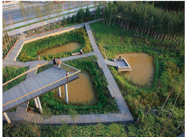
Figure 6.19: Terraced Biofiltration Ponds. These ponds at the Qunli National Urban Wetland captures and slows stormwater runoff (Turenscape N.D.).
