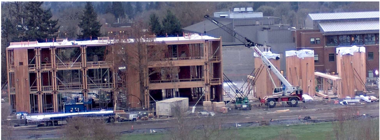
Figure 5-2: Peavy Hall Under Construction (Oregon State University, 2018)
