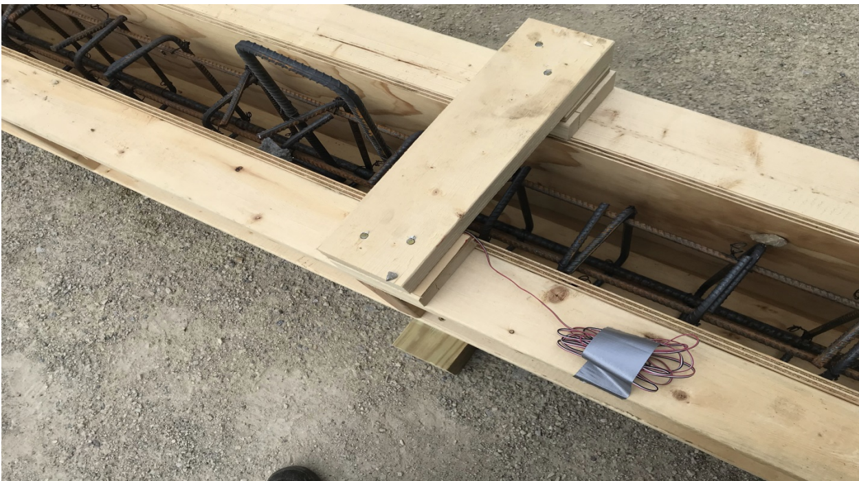
Figure 6-11 Form work and cage work with strain gages
