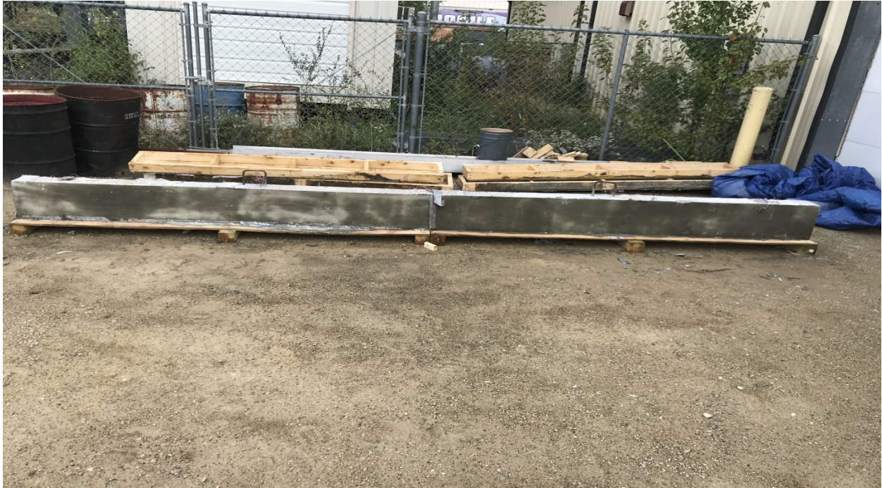
Figure 6-12 Casted reinforced concrete beam (front view)
