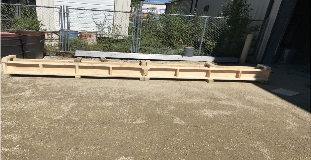
Figure 6-5 Form work (front view)
