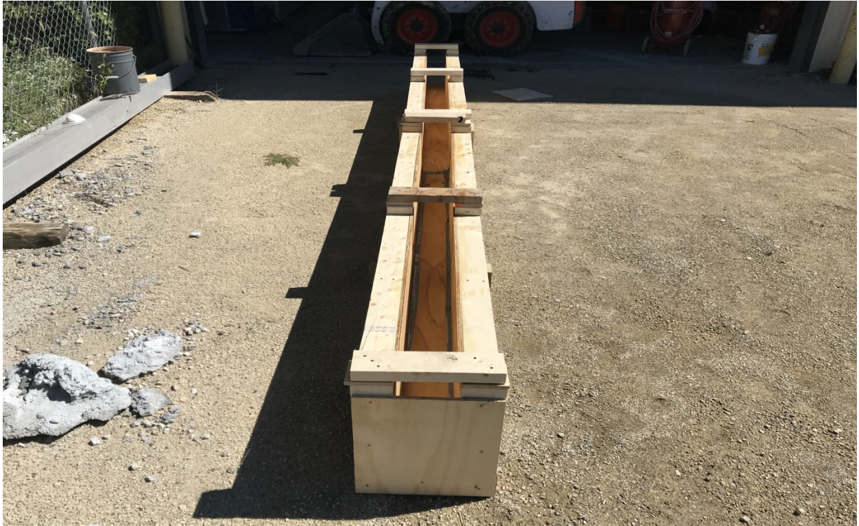
Figure 6-7 Form work (side view)
