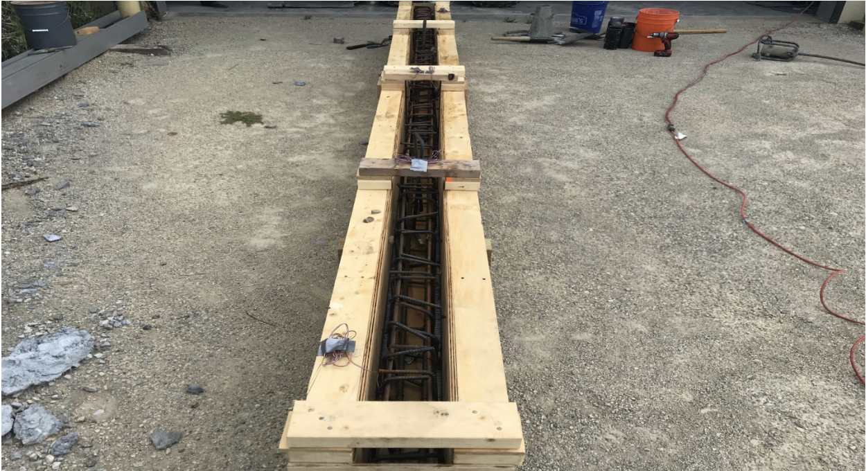
Figure 6-10 Form work and cage work
