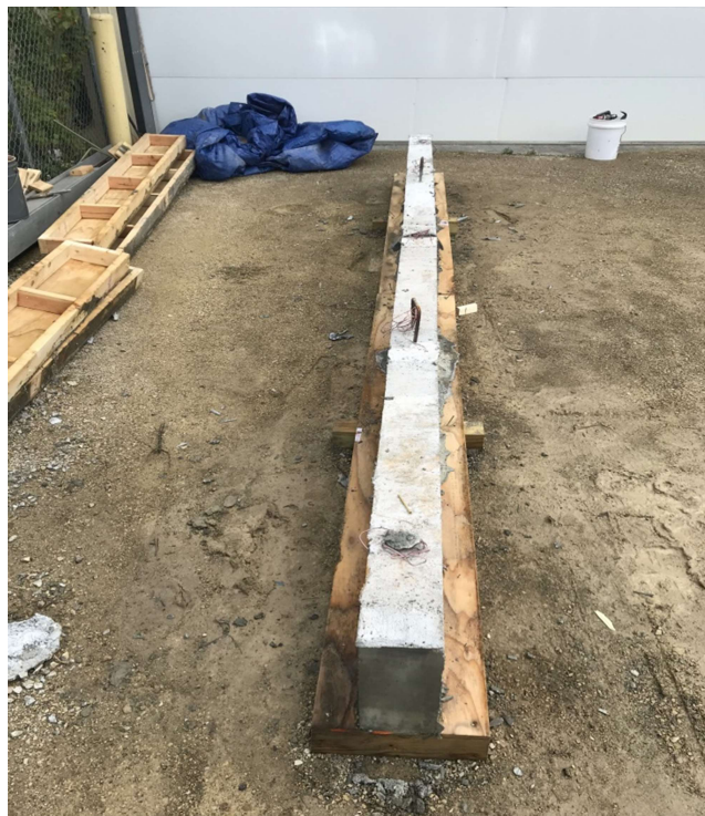
Figure 6-13 Casted reinforced concrete beam (side view)
