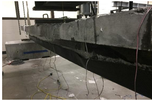
Figure 6-32 Beam T4 after the failure
