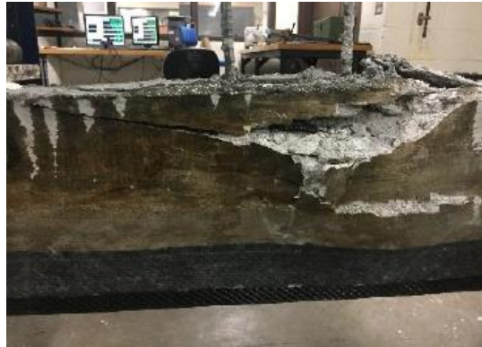
Figure 5-34 Beam R3 after the failure
