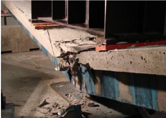
Figure 5-14 Failure of the beam T5 with U-wrap anchorage
