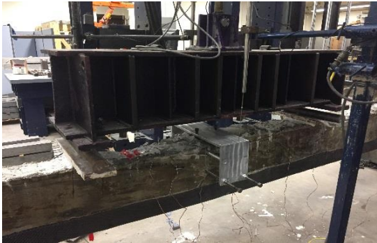
Figure 7-36 Beam R6 after the failure
