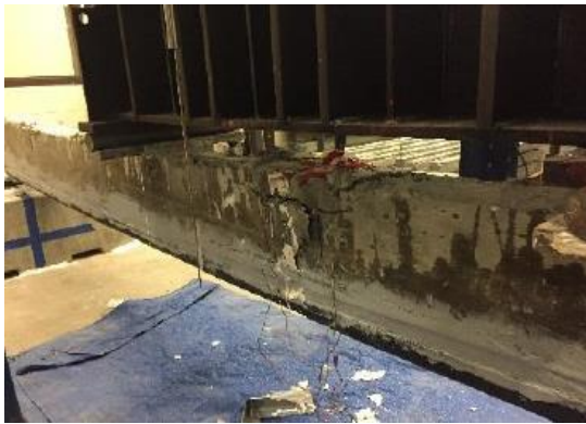
Figure 5-28 Beam R2 after the failure
