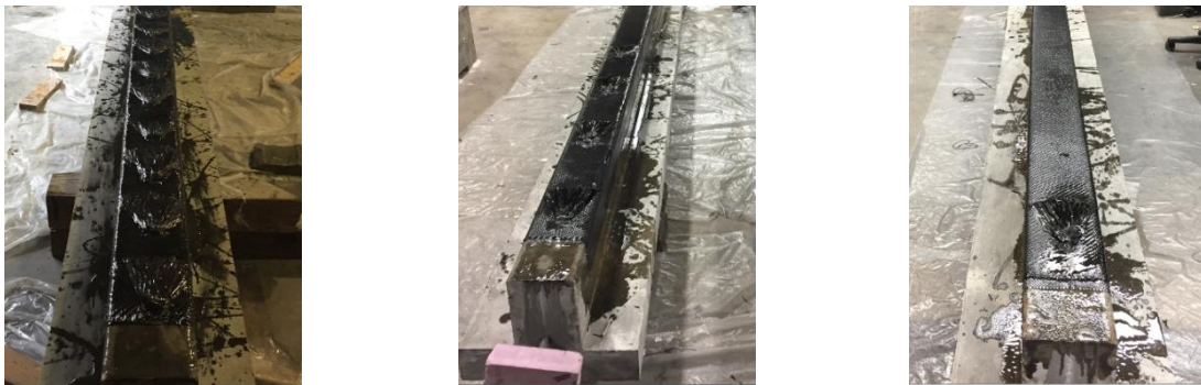
(a) (b) (c) Figure 6-11 Application of CFRP sheets and anchors (a) beam T3; (b) beam T4; (c) beam T5
