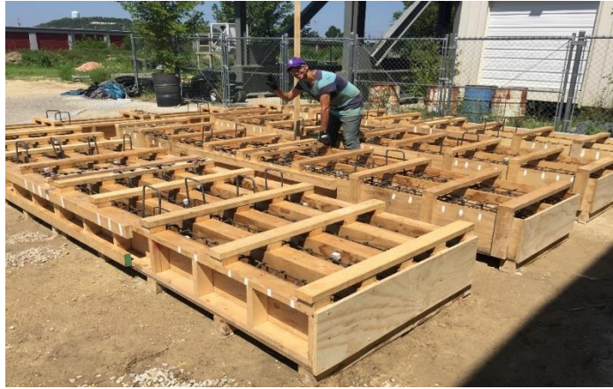
Figure 4-4 Placing the spacers
