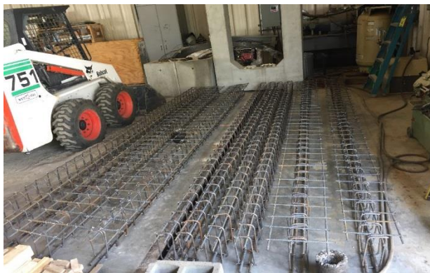
Figure 4-2 Rebar cages for the T and rectangular beams
