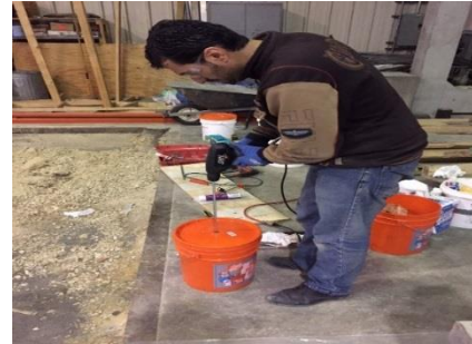
Figure 3-6 Mixing the epoxy
