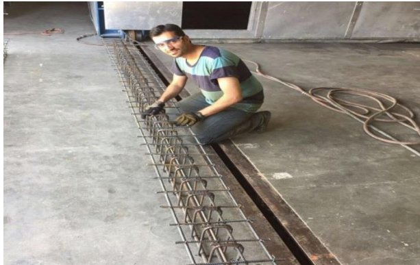
Figure 4-1 Fabricating the steel rebar caging
