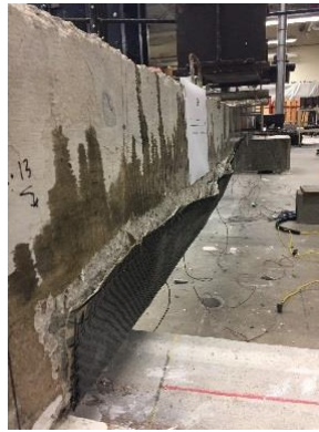
Figure 7-43 Beam R7 after the failure
