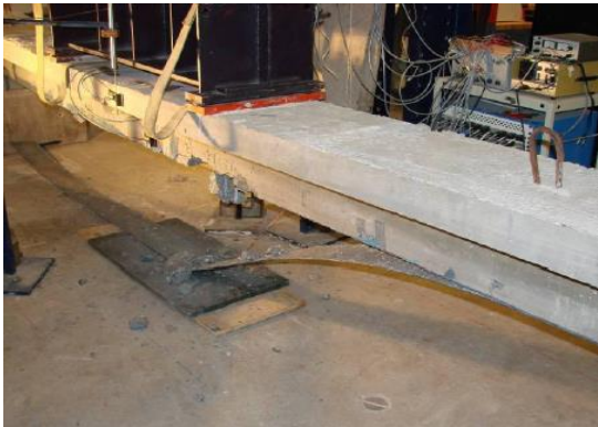
Figure 5-13 Beam T4 after the failure
