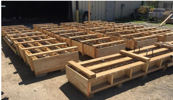
Figure 4-5 Getting ready to cast the concrete
