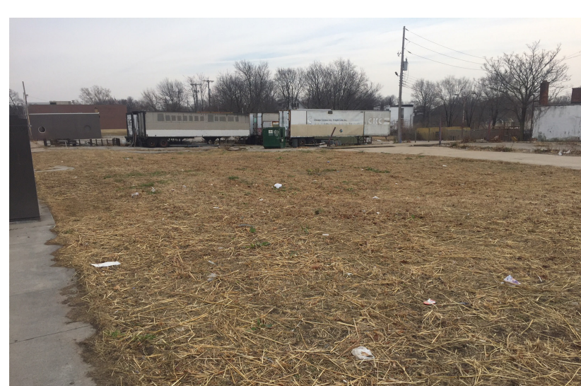
Figure 14. Weeds growing through cracked pavement on the site.
