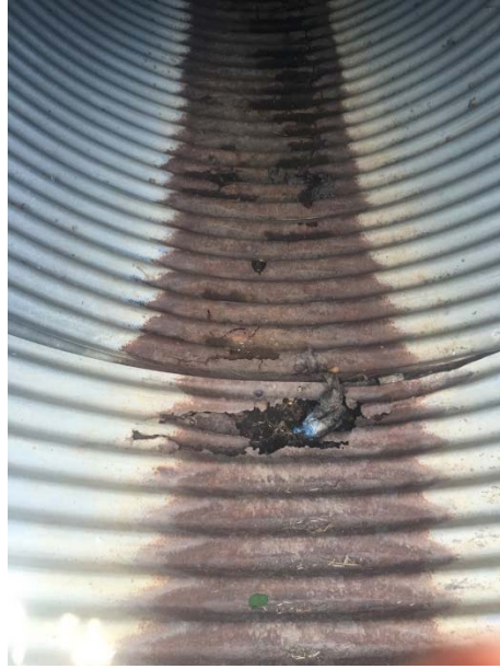
Figure 4-5: Severe Invert Corrosion under Dry Conditions
