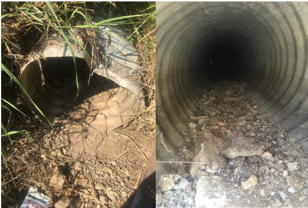
Figure 4-3: Example CMPs with Non-Corrosion Induced External Damage and Invert Silting
