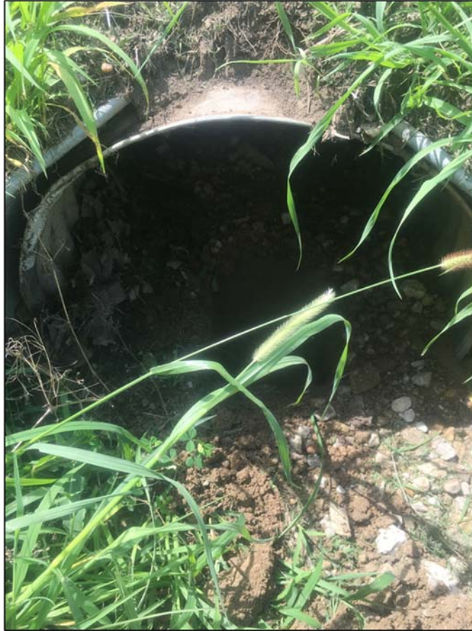
Figure 3-1: CMP with Heavy Invert Silting
