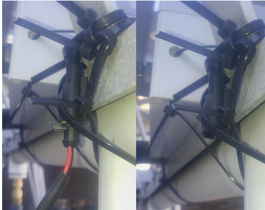
Figure 18. Wires connecting the drop hose to the sprinkler node connected (left) and disconnected (right) while testing the detection of detached drop hoses.
