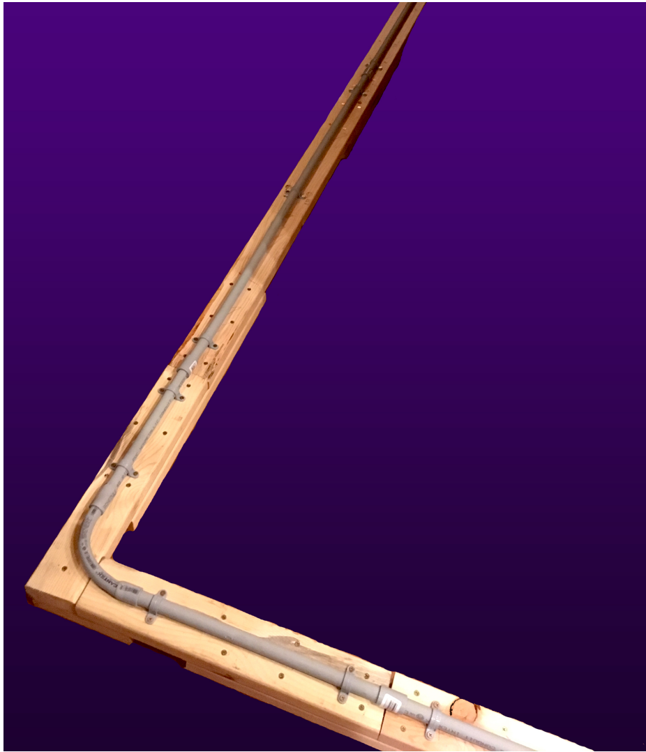
Figure 3-1: Conduit Construction with a Factory Elbow Connecting Two Conduit Legs
