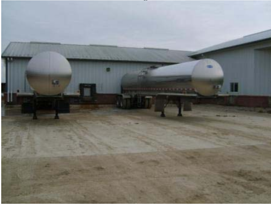
Figure 5.3: DTL Barn with Concrete Loading Slab
