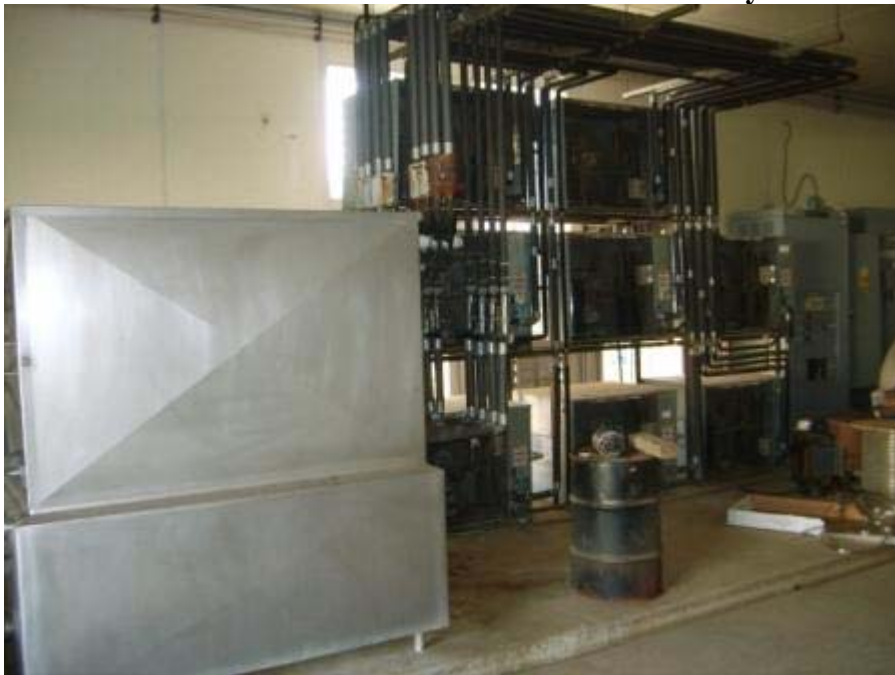
Figure 5.5: Cabinet Chiller and Bank of Condensers for a DTL System
