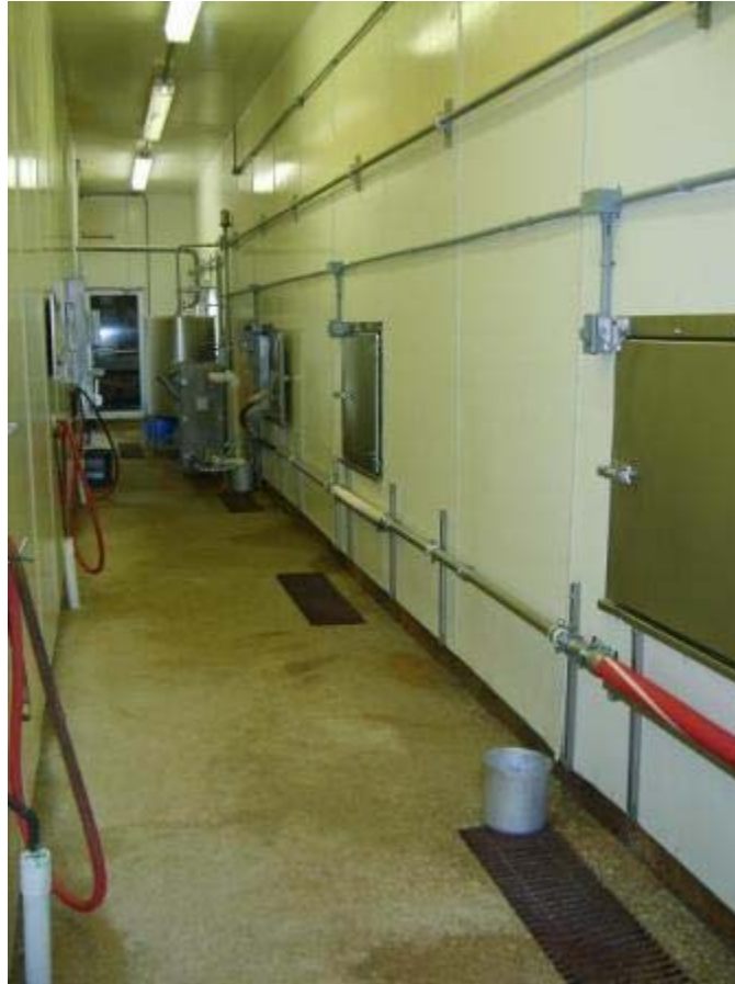
Figure 5.2: DTL Load out Doors
