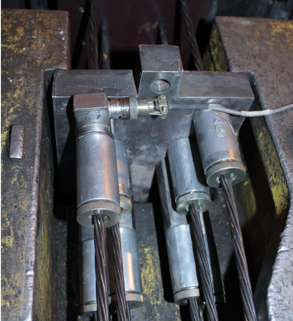
Figure 89 A center-hole load cell was installed on one of the tendons at the live end to verify the correct prestressing force was achieved with the special jacking plate apparatus
