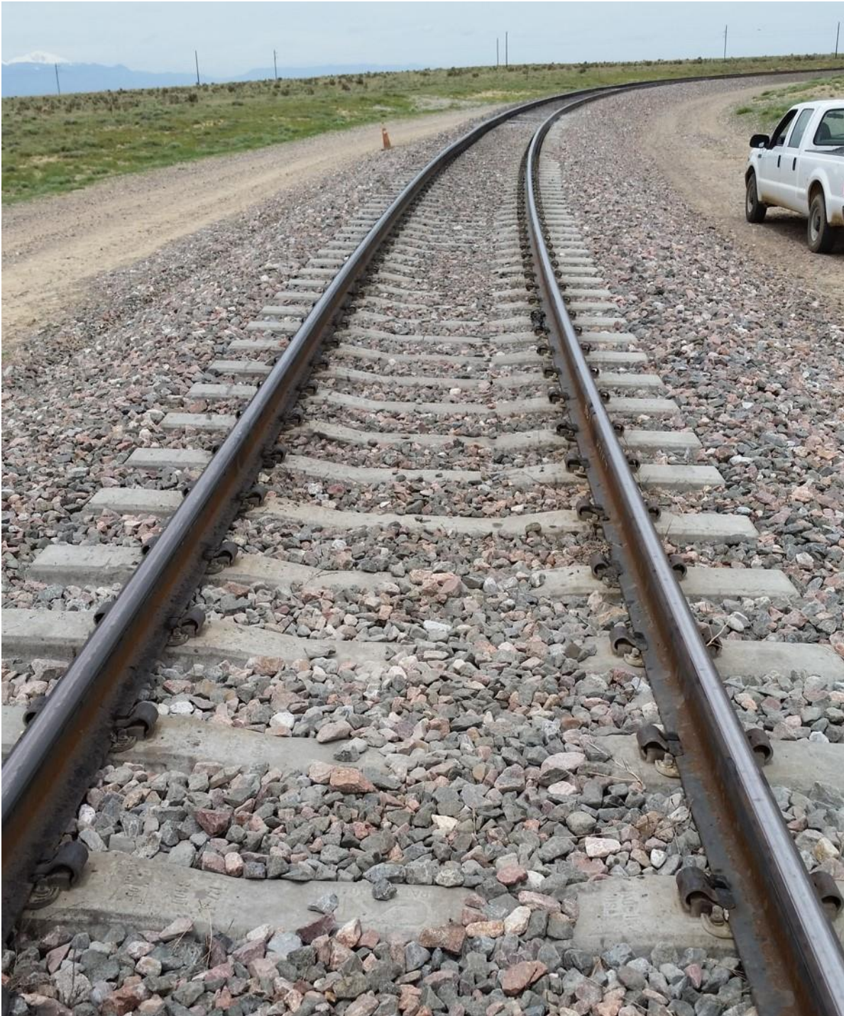
Figure 127 “T”-marked crosssties installed in curved track during Stage III
