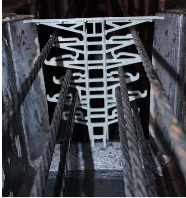
Figure 79 Wire chair used to support 3/8-in.-diameter 7-wire strand
