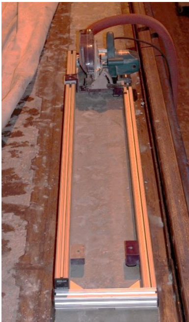
(a) Track-mounted saw used to cut groove
