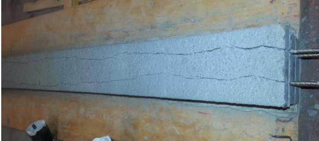
Figure 64 Severe longitudinal splitting occurred along the [WH] wires in prisms cast with Mix-Design #2
