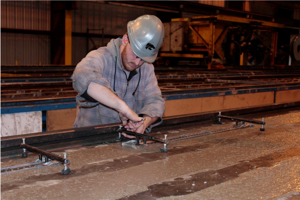
Figure 94 Steel bars used to hold brass inserts at proper spacing in the concrete crossies
