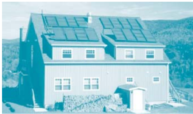
Figure 2.4 Thermal Collectors at the Chanterelle Inn (Natural Resources Canada, 2002)
