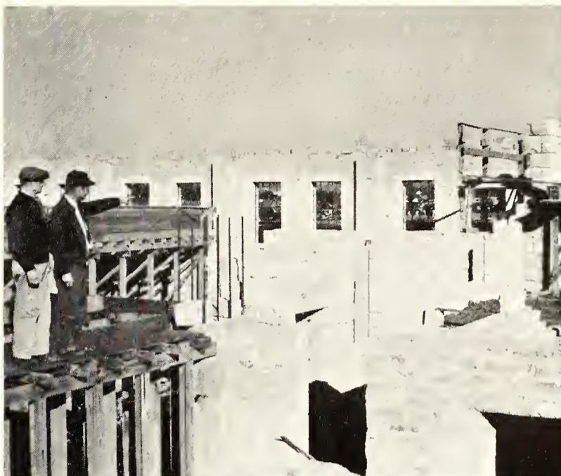
THE NEW MILITARY building takes form slowly as priorities and war industries hold up necessary material.
