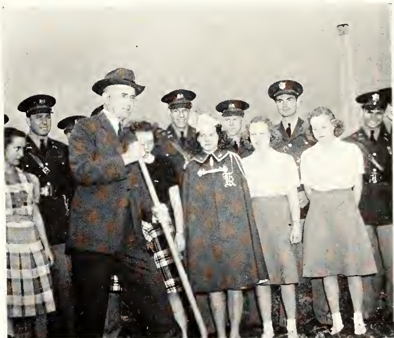
PRESIDENT FARRELL breaks ground for the new Military Science building.
