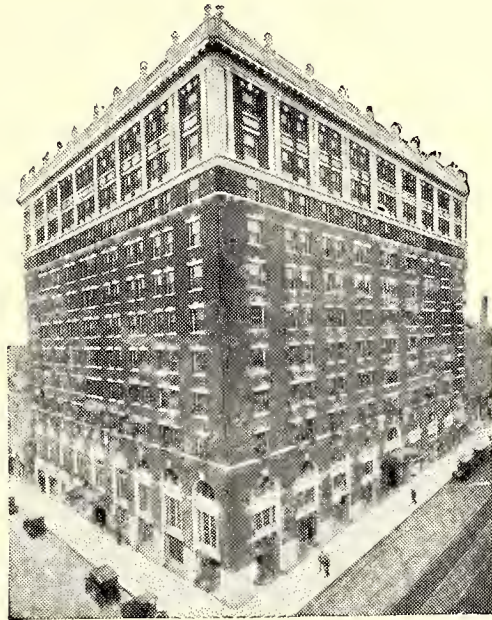
HOTEL MUEHLEBACH 500 ROOMS
