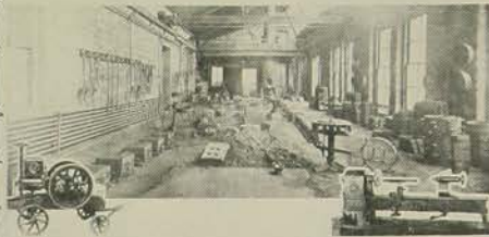
FABRICATOR'S WORKSHOP WITH VARIOUS MACHINERY
