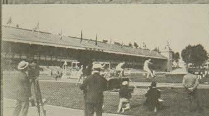
That caused water hazard
