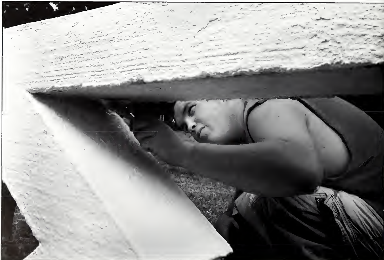
Coating the underside corner of the four and one-half foot "Sigma," Zach Stover, freshman in computer engineering, paints the concrete letters in front of Delta Sigma Psi Aug. 15. Members re-painted the house letters as part of preparing the house for the school year. (Photo by Karen Mikols)
