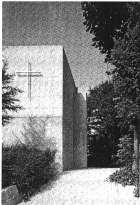
Exterior View of the Rear Opening Drew, 1996, P 24
