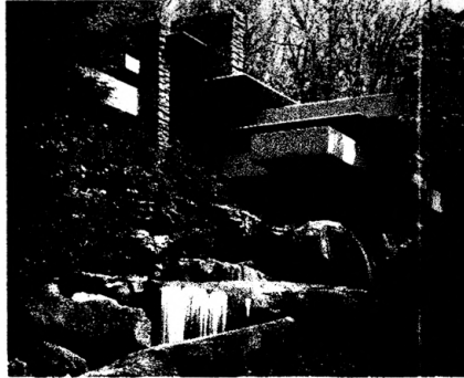
Figure 5.11. The horizontal course of stone masonry as a continuation of the rock ledges of Bear Run
