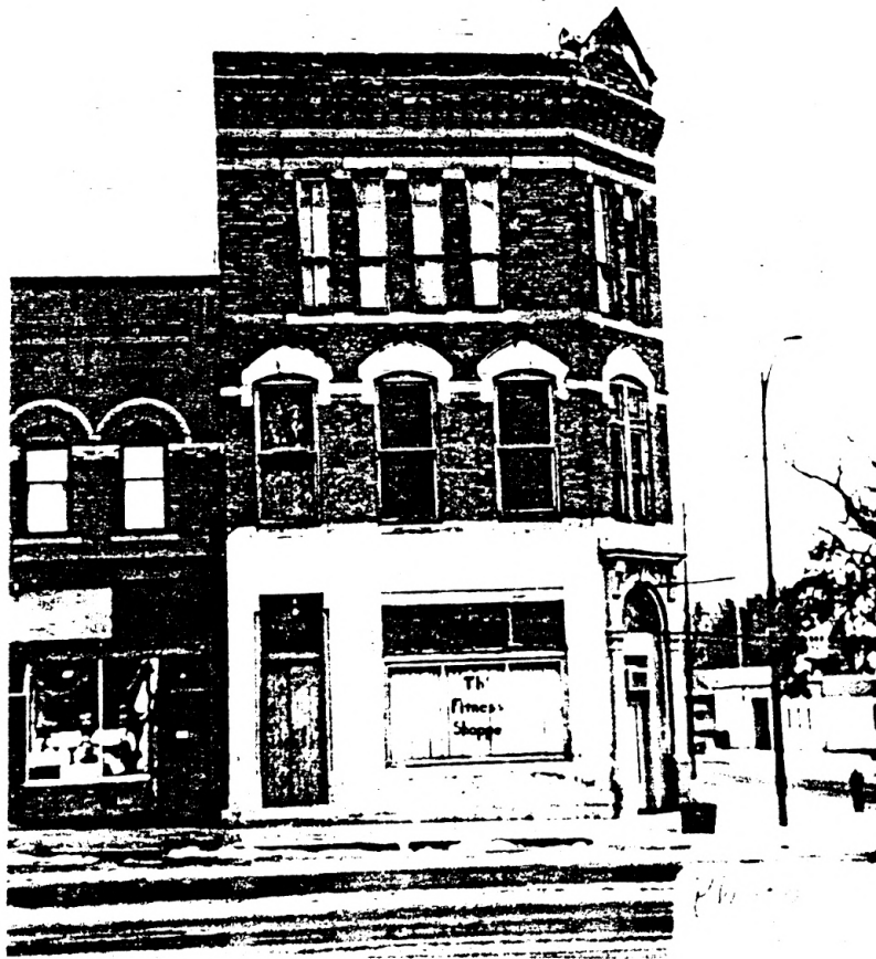
Photo 2-10 Existing Exterior Condition (South Facade) (Photo taken by Lichang Jin in January 1991)
