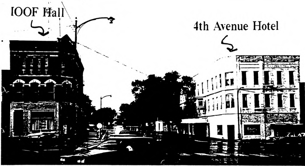
Photo 2-3 (above) The IOOF Hall, 4th Avenue Looking East Photo 2-4 (below) The IOOF Hall, Oak Street Looking North
