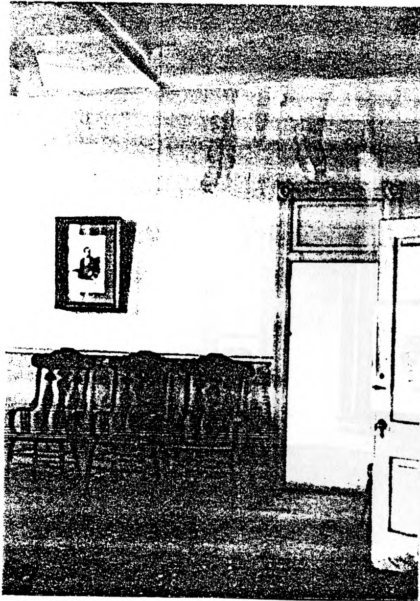
Photo 2-27 Existing Interior Condition - 2nd Floor, Space #9 (Photo taken in January 1991 by Lichang Jin)
