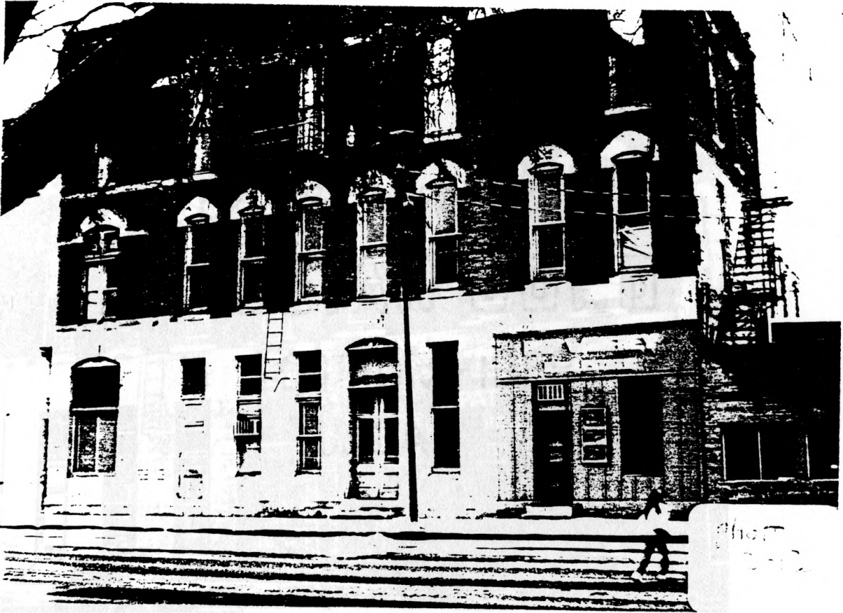
Photo 2-12 Existing Exterior Condition (East Facade)
