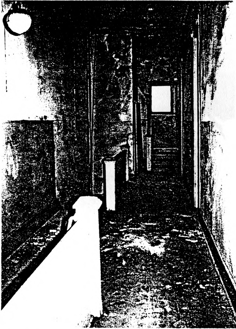
Photo 2-22 Existing Interior Condition - 2nd Floor, Space #7 (Photo taken in January 1991 by Lichang Jin)
