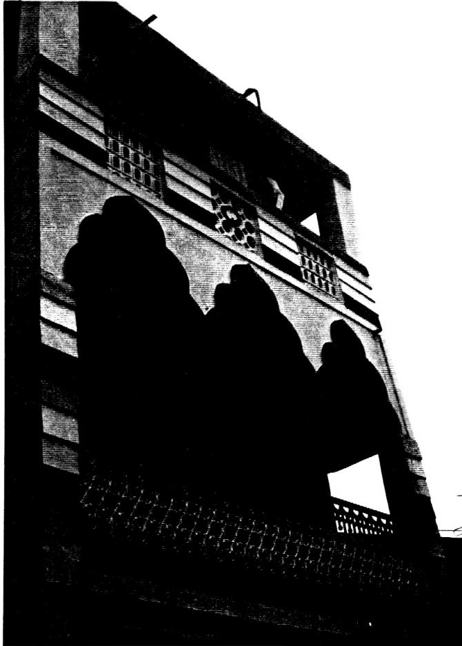
Fig. 5.17: HOME IX Second floor balcony facing street below
