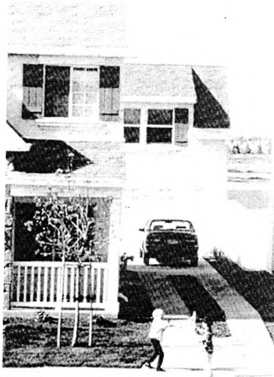
Figure 5.20 Rear Garage in Laguna West
