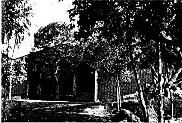
Fig. 4.41 The stark, bare exterior of the Loyola Chapel.
