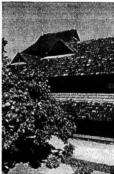
Fig. 2.4 The Padmanabhapuram Palace.
