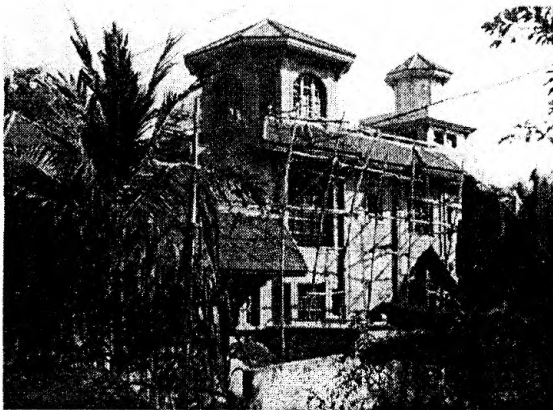
Fig. 2.13 A return to gimmicky 'tradition'; concrete roofs capped with tiles and depthless, elevational arches.
