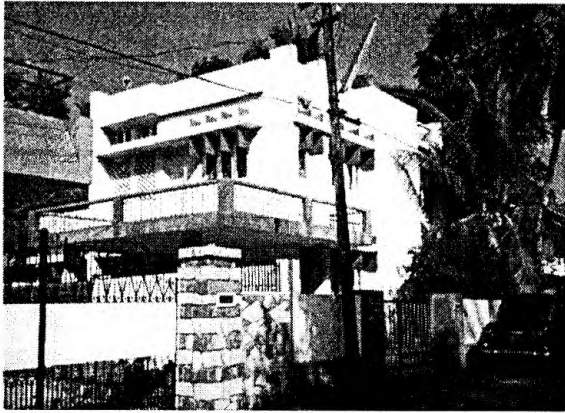
Fig. 2.12 A residence in Trivandrum, Kerala: Attempts at Modernism and Corbusier'ian shading elements.
