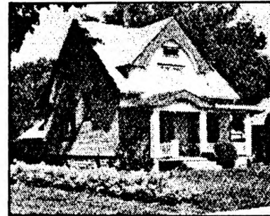
House In Lindsborg. It is said to have the first flush toilet in town! (Smoky Valley Historical Association.)
