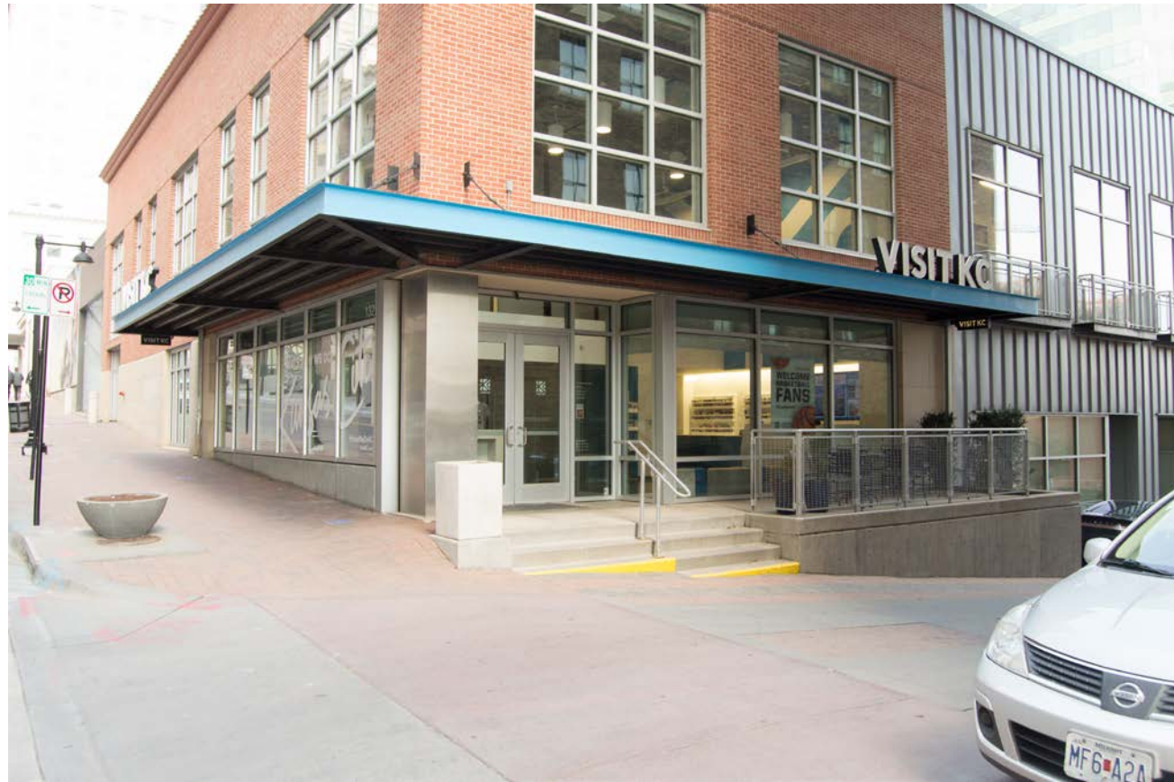
The Power & Light District houses two public communicational facilities. The first being the Public Safety Office (see figure 4.66) and the VisitKC offices on the Western border of the Power & Light District.
