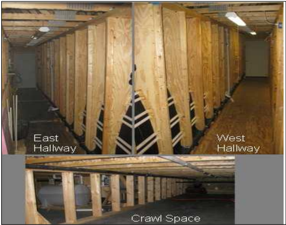
Figure 3.2 East and West Hallways and Crawl Space (Beneke, 2010)
