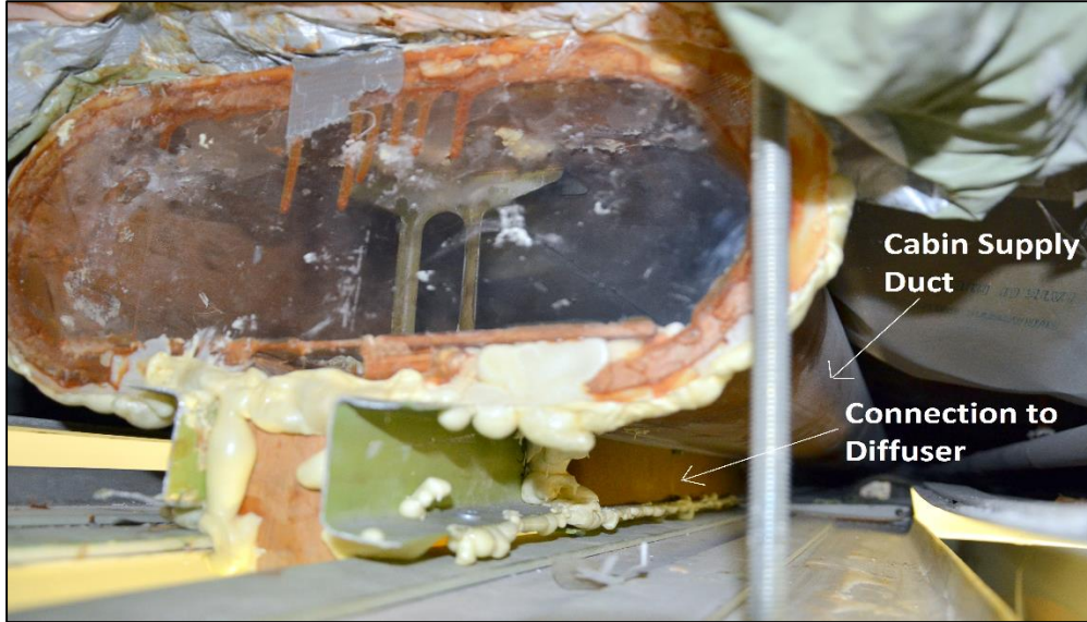
Figure 3.20 Boeing 737 Cabin Supply Duct with Connection to the Diffuser
