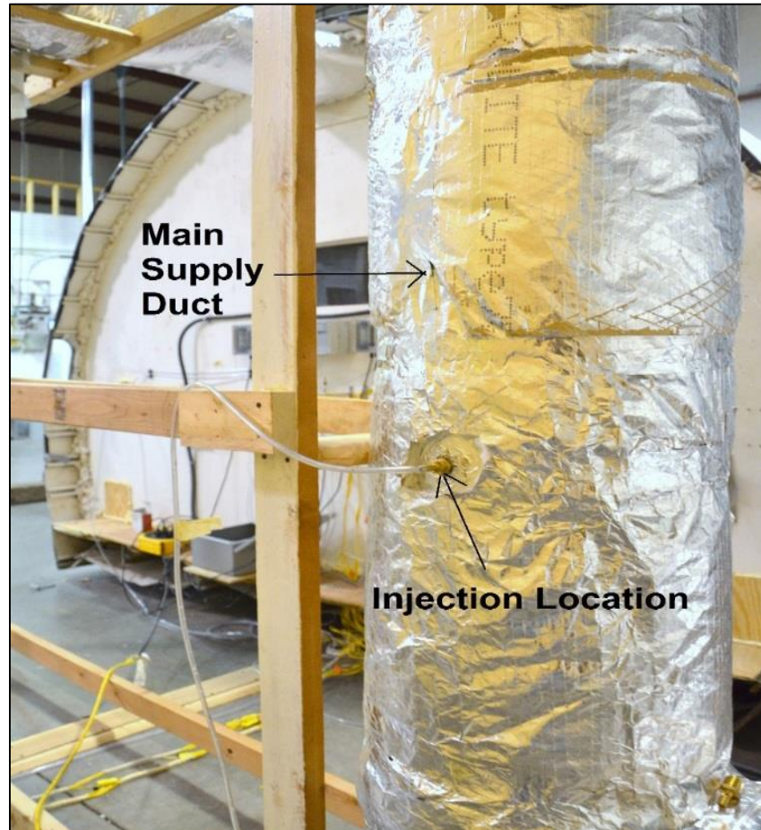
Figure 4.1 Tracer Gas Injection Location For Ventilation Effectiveness Study
