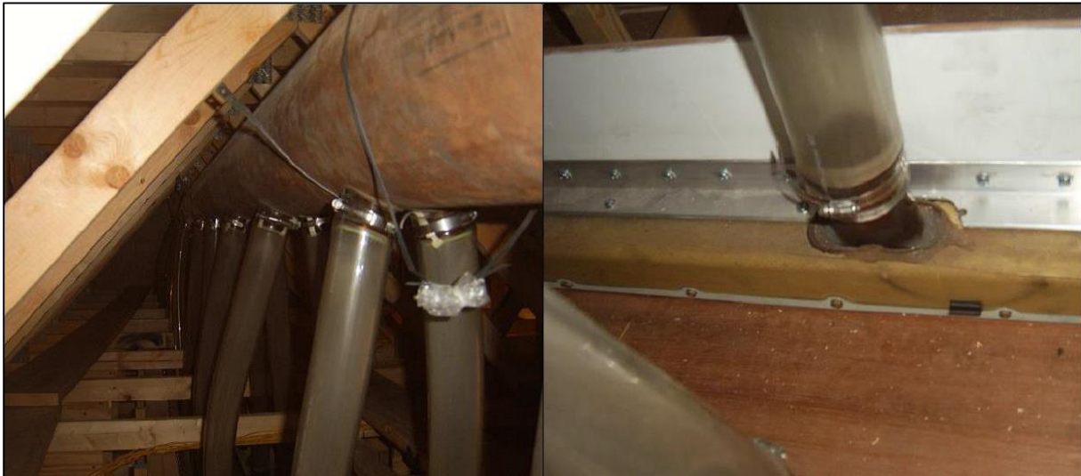
Figure 3.19 Boeing 767 Cabin Supply Duct with Flexible Tubes Connected to Diffuser
