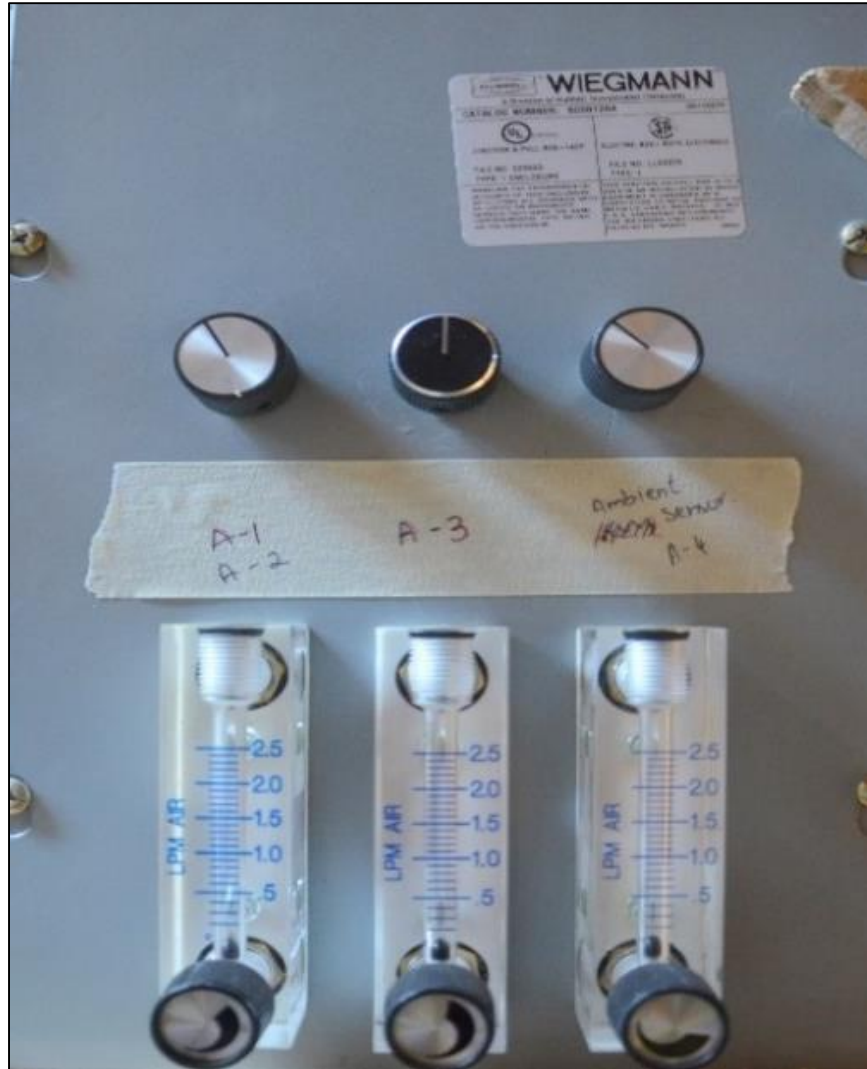
Figure 3.27 The Flow Balancing System
