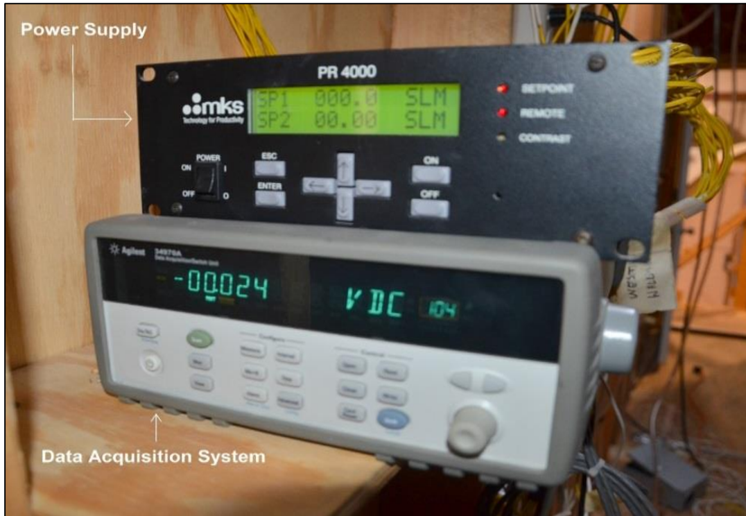
Figure 3.28 DAQ System Along With the Power Supply
