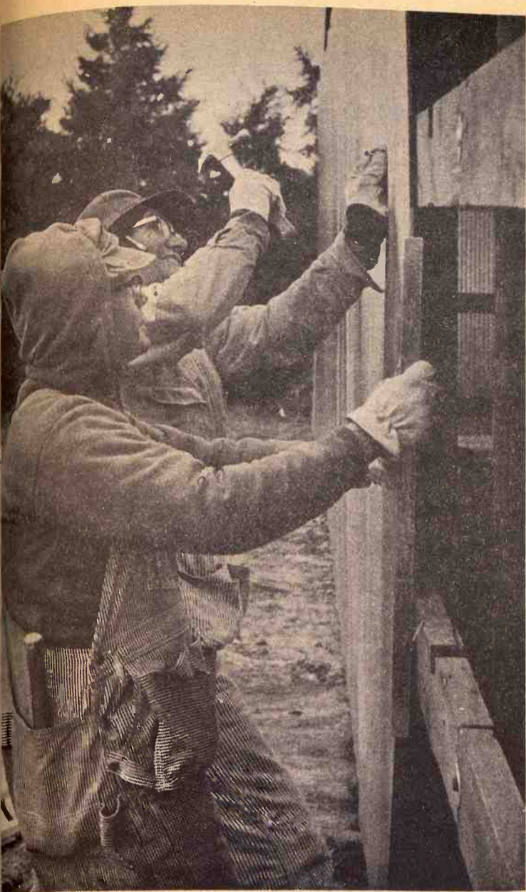
NEW MACHINE SHED Dennis Cooley (left) and Arnold Swanson of Gypsum are shown here building a new machine shed on the James Pettie farm south of Gypsum. Part of the material was salvaged from a shed that was blown down last June.
