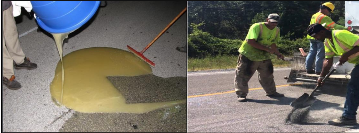
Figure 2.9 HFST manual application (HFST overview, FDOT, 2015)
