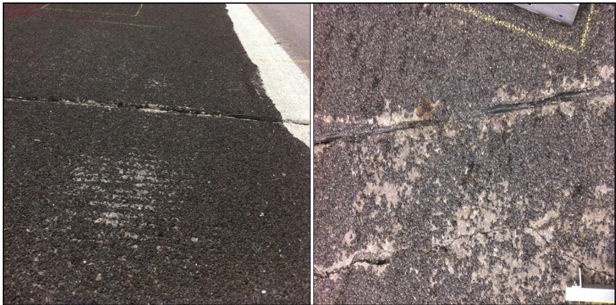
Figure 2.21 De-bonding of high friction surface aggregates
