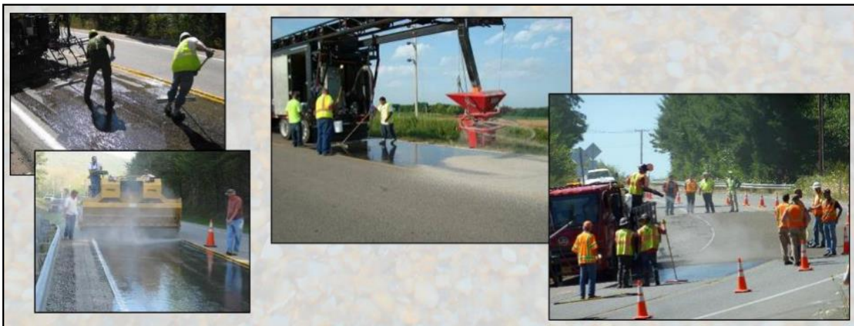
Figure 2.10 HFST semi-automated application (HFST overview, FDOT, 2015)
