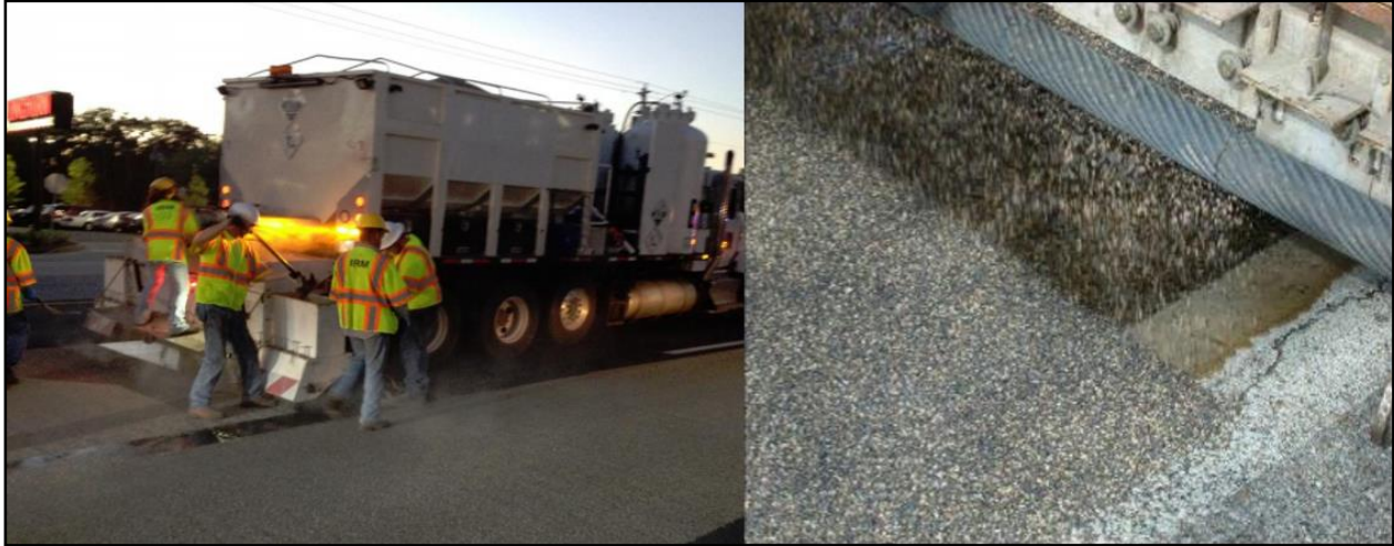
Figure 2.11 HFST fully automated application (HFST overview, FDOT, 2015)
