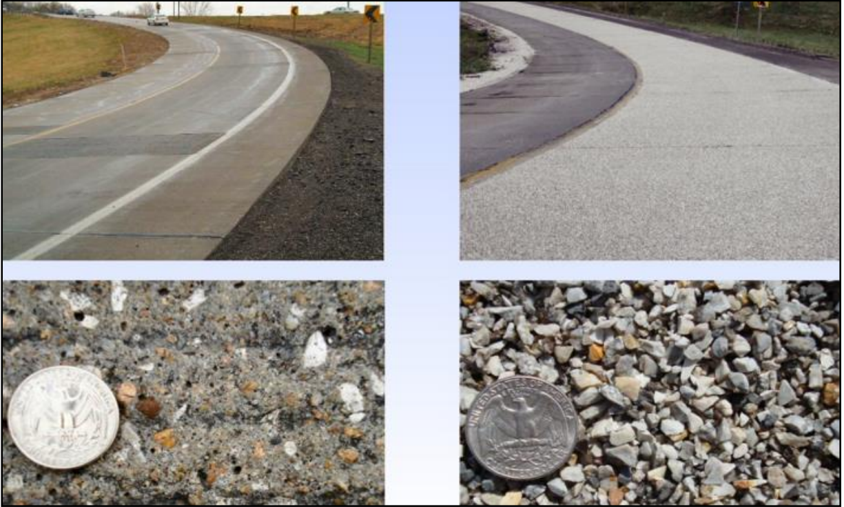
Figure 2.18 Before and after HFST on I-35/I-635 ramp in Kansas City (concrete pavement)
