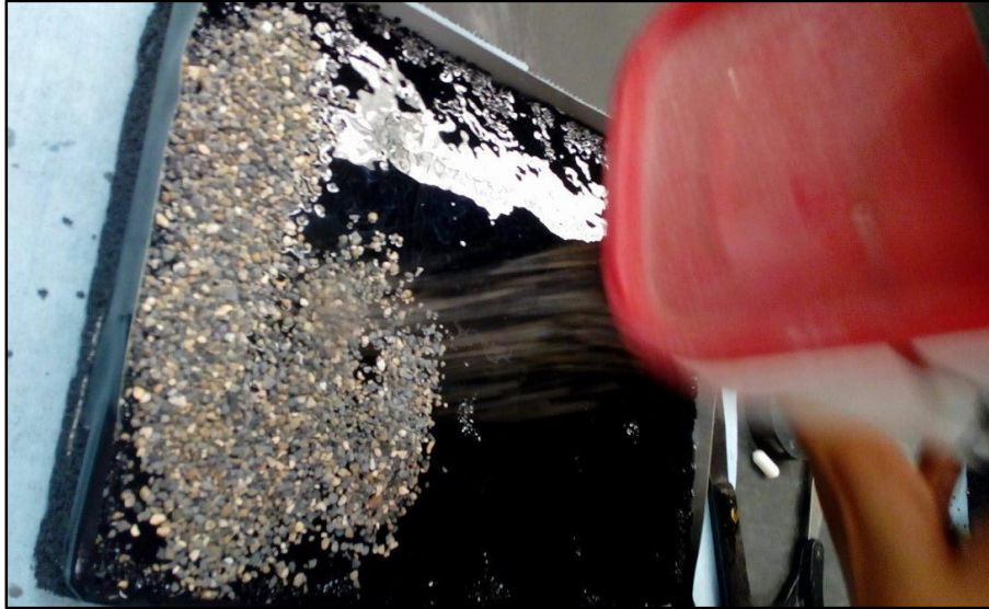
Figure 3.16 Aggregate is being spread over the epoxy covered slab
