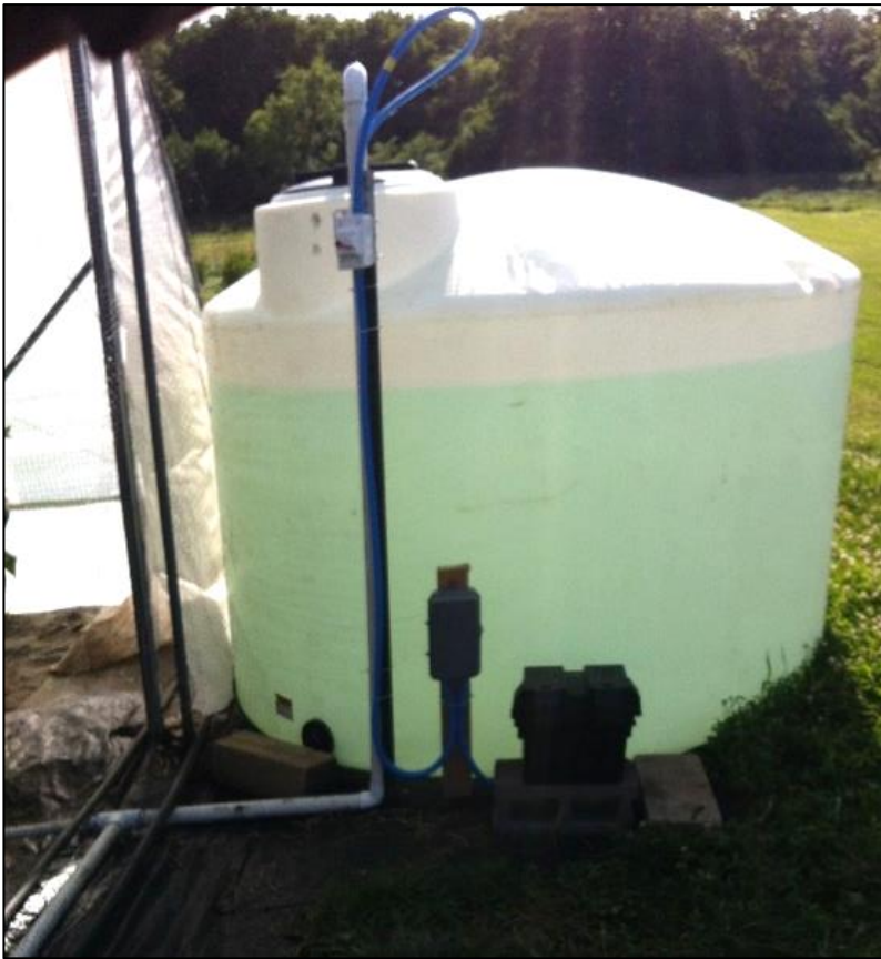
Figure 2- 1000-gallon tank situated at the north end of the high tunnel that held water for the evaporative cooling applications.
