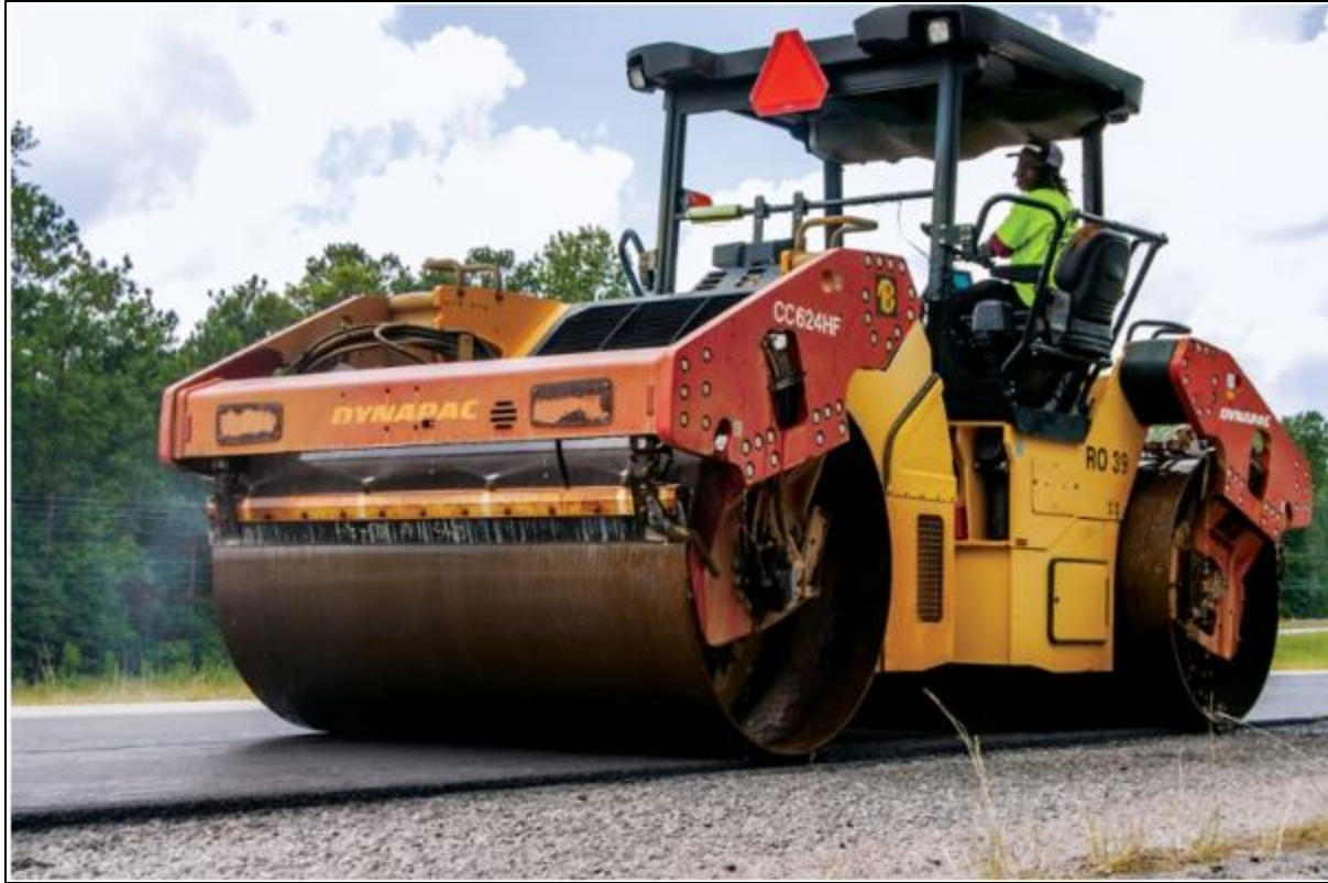
Figure 6-6 Compaction of an HMA overlay (National Center for Asphalt Technology b )
