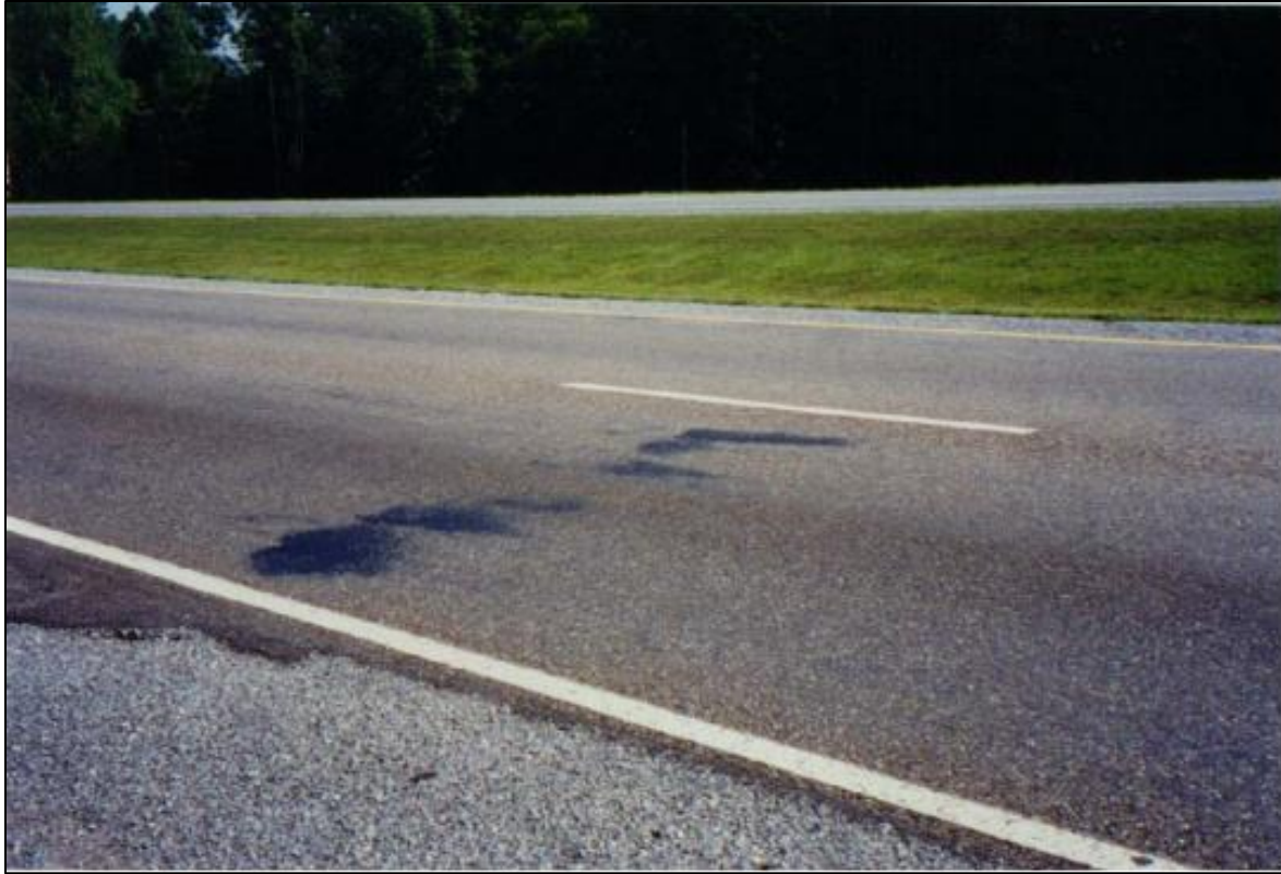
Figure 6-7 UBAS layer on top of existing asphalt pavement surface (Kandhal and Lockett 1998)
