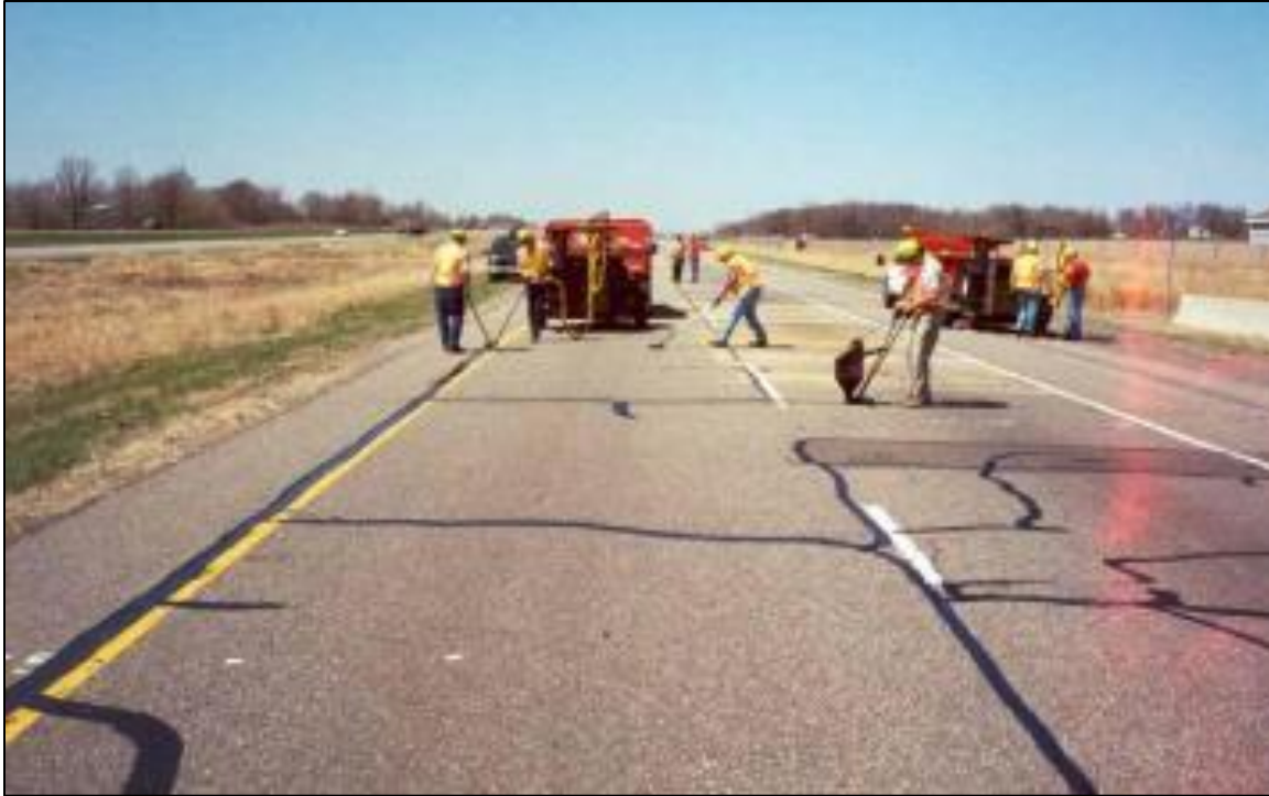
Figure 6-1 a) Crack treatment operation on HMA pavement (Minnesota Maintenance Manual 2014)
