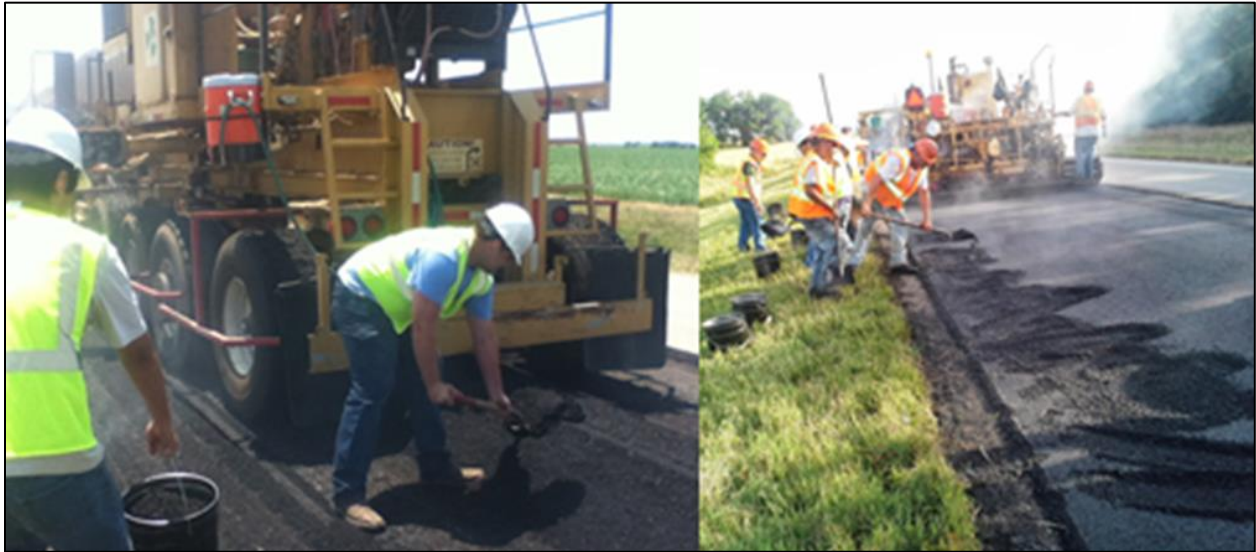
Figure 3-2 HIR sample collection in front of (left) and behind (right) the paver
