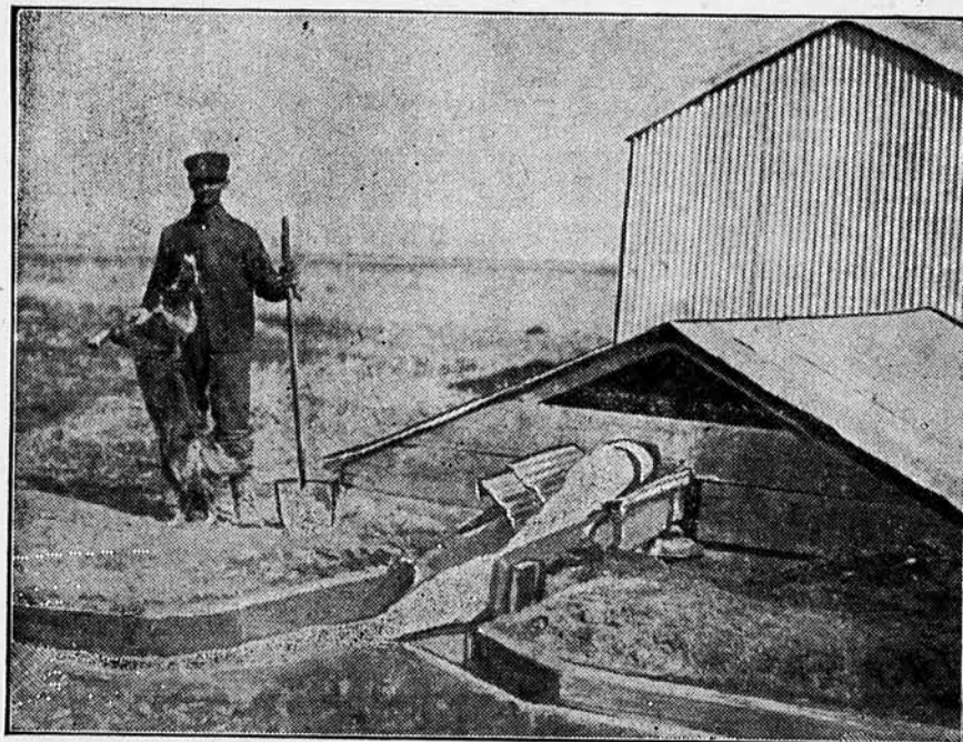
Water leaving a 7-inch pipe from M. L. Dickson's pumping irrigation plant in Clark county, probably the first of its kind in the Cimarron Valley. The pump, and 12 horsepower kerosene engine lifts 700 gallons a minute. Mr. Dickson, though not an expert, installed the plant himself. Elsewhere on this page he describes how the work was done.
