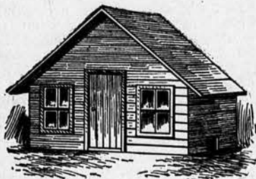
Fig. 1.—Implement house transformed into poultry house.
