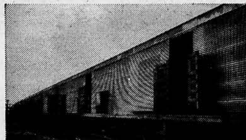
Double-deck stock loading platform viewed from trackside, having floor-level and stair-step ramps at each door.
