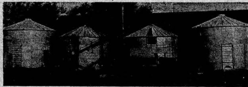
THIS IS EQUIPMENT that speeds harvest for George Rush. Grain in one bin is dried while the other is being filled. When moisture is lowered to 14 per cent, batch is transferred into permanent storage. Dryer unit and fuel tank are in front of third bin from left.
