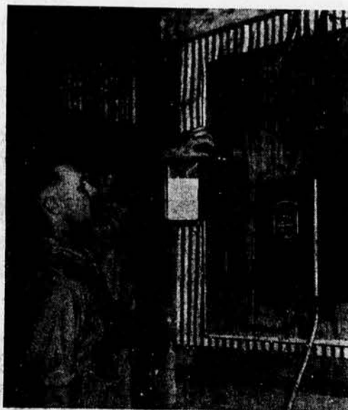
BLOWERS FOR CURING HAY in the French hay barn are controlled by a magnetic switch timed by a clock that allows 2 "ons" and 2 "offs" each 24 hours.
