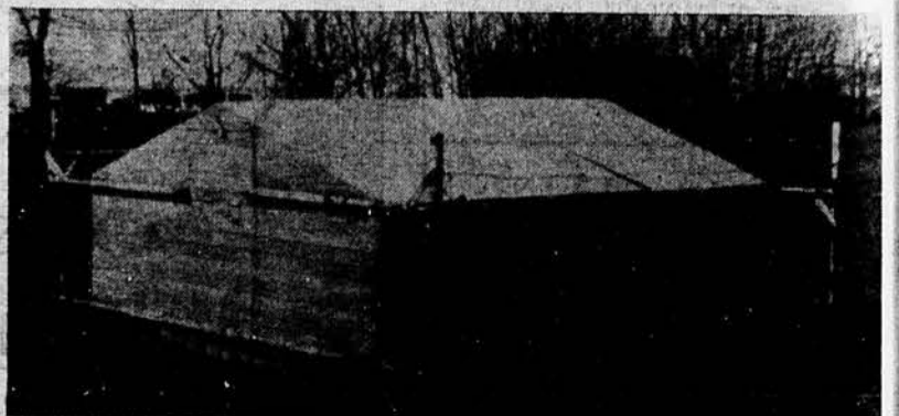
METAL FRAME on this creep-feeder, built by Harold McDonald, Anderson county, telescopes against the frame center so it will go thru gates easier and so size of creep entrance can be easily adjusted.
