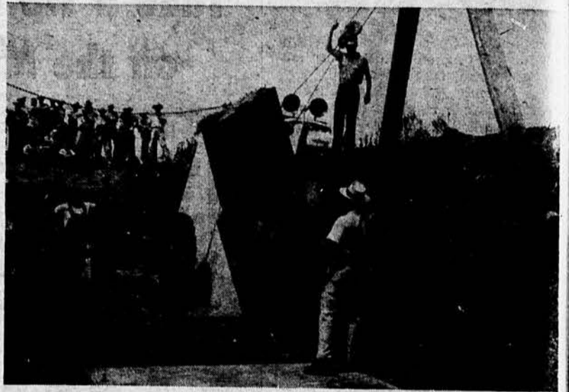
TILT-UP SILO going into place on Wayne L. Knopp farm, south and east of Chapman, is part of silage field day held July 21. Knopp stands on bank at right, directing lifting of concrete slab that was poured on silo floor. Leo Wendling, Kansas State College Extension engineer, holds block behind slab to position it correctly as A. R. Schmidt, a neighbor, stands by tractor he used to slide base of slab. Keller Gordon of Portland Cement Association stands at extreme left with camera at eye level.
