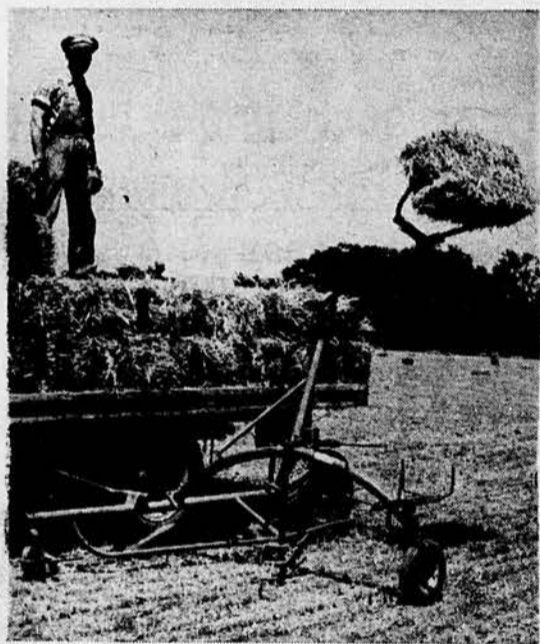
A BIG LABORSAYER is this new-type baled hay loader being used by Tom Holmes, Garnett.
