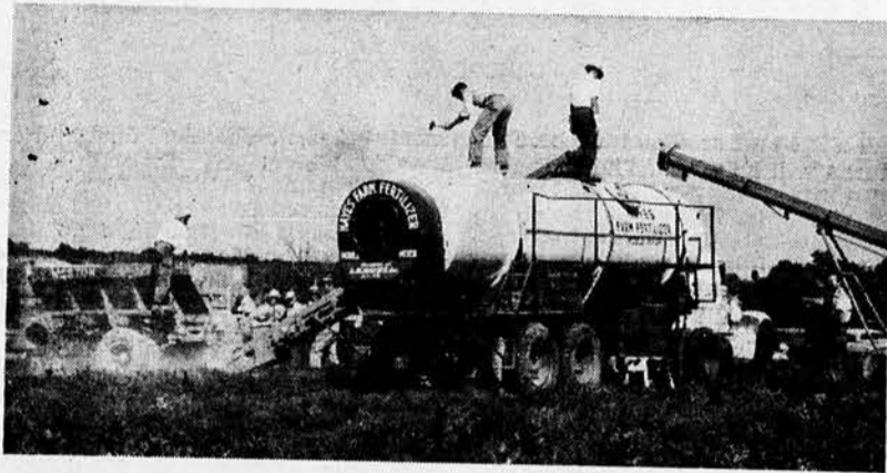
MOBILE MIXER: Limestone from the truck at left is being elevated into the mixer barrel. Phosphate, potash if needed and ammonium sulphate were put into the mixer thru the elevator at right. After all fertilizer components are in the huge barrel, it revolves to mix the goods much like a concrete mixer. Spiral vanes inside the barrel move fertilizer forward. Then the drum is reversed to move the mixture back.
