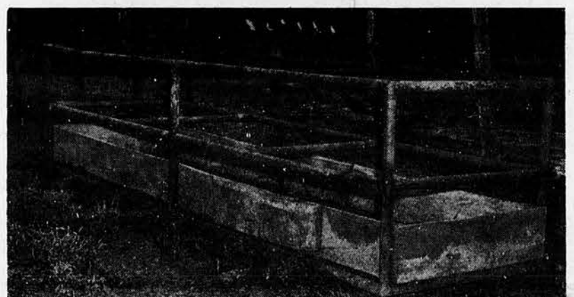
SKID BUNKS like these are made in the Elwood King farm shop, Butler county. Bunks are 4 by 16 feet and are used for silage and hay. Kick boards are of native lumber.
