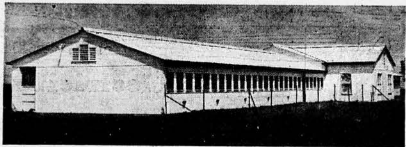
POULTRY BUILDING at Moorman Experimental Farm, Quincy, where Moorman company has extensive tests for its products. This farm attempts to simulate conditions found on the average farm.
