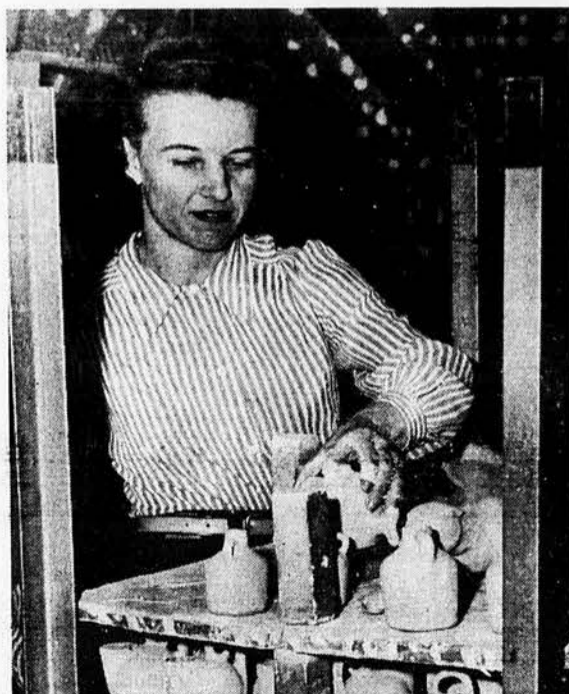
Mrs. Don Hokr arranges pottery on racks for putting into the kiln. Glazed pottery has to be baked before and after glazing.
