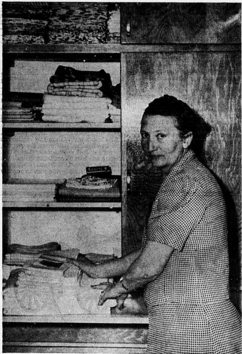
This linen closet has a disappearing service counter, being demonstrated by Mrs. Ben F. Jerman, Seward county. She can put her armload of linens on the counter while filling the shelves, then push the counter back into the cabinet out of the way.
