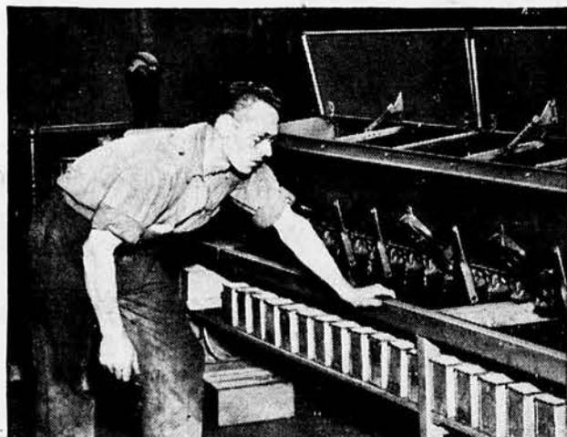
McCormick drills are grain-tested at the factory to make sure that each fluted feed cup meters out seed at the same, even rate, and that the drill as a whole will seed at the rate you set it for. No over-planting, no under-planting.
