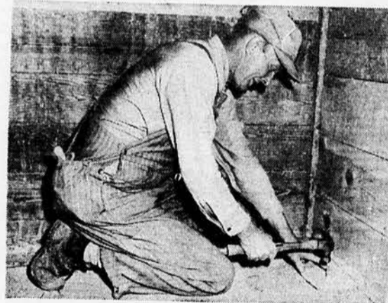
TIGHT BIN SAFEST: Mr. Doebert covers a hole in the bin floor by nailing down a board over the opening.
