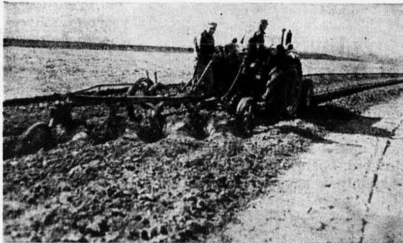
ON THE JOB: This picture was taken on the second terrace after the individual classes were started on their respective terraces. The tractor is a 55 Massey-Harris pulling a 4-bottom, 16-inch plow. The driver is Ferd Haukap, the rider is Marion Mooberry.
