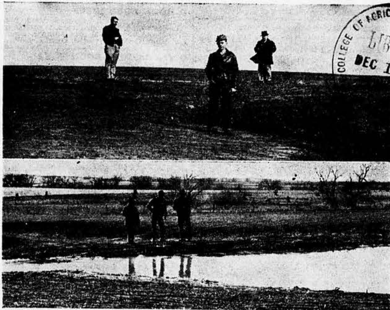
These pictures give 2 views of one gully-stopping operation which Kurtes Blomquist performed the first year of the county program. Top photo was taken below the terrace. Blomquist is standing in the center where there was a ditch large enough to hide a tractor. On top the terrace at left is County Agent Charles Pence, at right, Jay Payne, district work-unit leader. Lower photo was taken from the other side of the same terrace. It shows not all water drained out of the depression at first. But it was silting in and would fill completely in time.
