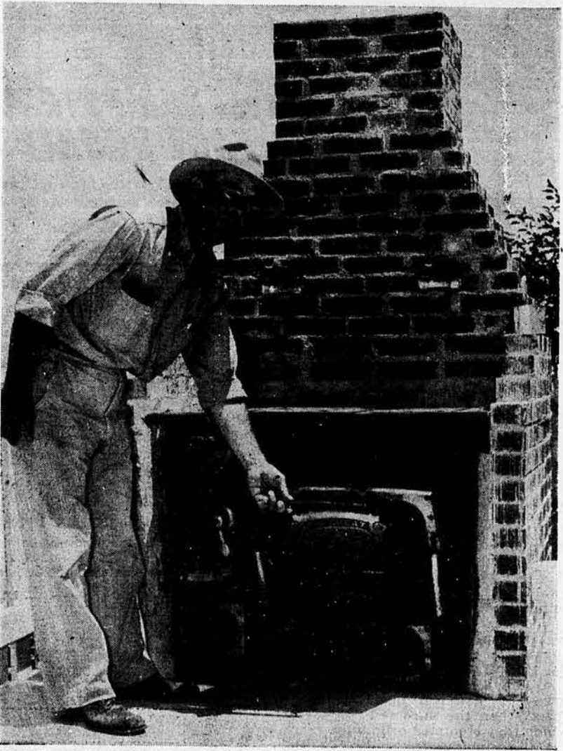
A discarded wood-burning kitchen range makes an excellent outdoor fireplace when properly installed. This one on the Jess Taylor farm is being demonstrated by Mr. Taylor.
