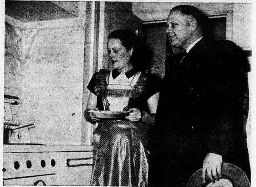
In the Neff home, electricity plays a big part. Much of the electrical equipment was installed under the supervision of Lee King, Kansas Gas and Electric Company rural representative, shown here with Mrs. Neff.
