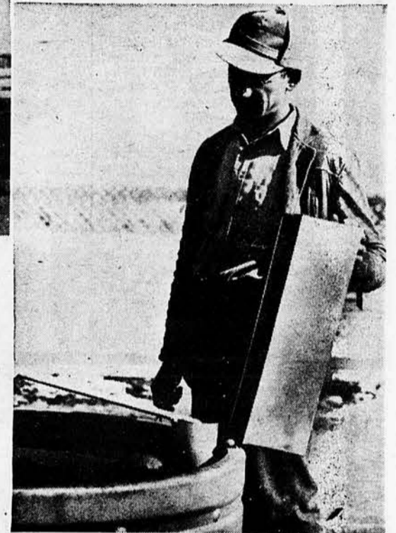
Above: Metal box which protects tank's float-control mechanism is hinged to side of tank. Here Mr. Byler holds it open. Flue from heat chamber below is next to rim of tank. In addition to protecting the float, this metal hood disperses heat from below around the float area. During exceptionally severe weather, ice might form at edges of tank, but not around float. In this tank water can be kept at 50 degrees with little difficulty. That means more milk because dairy cows require more water in winter than in summer. Cows do not perspire, get water from green pastures.
