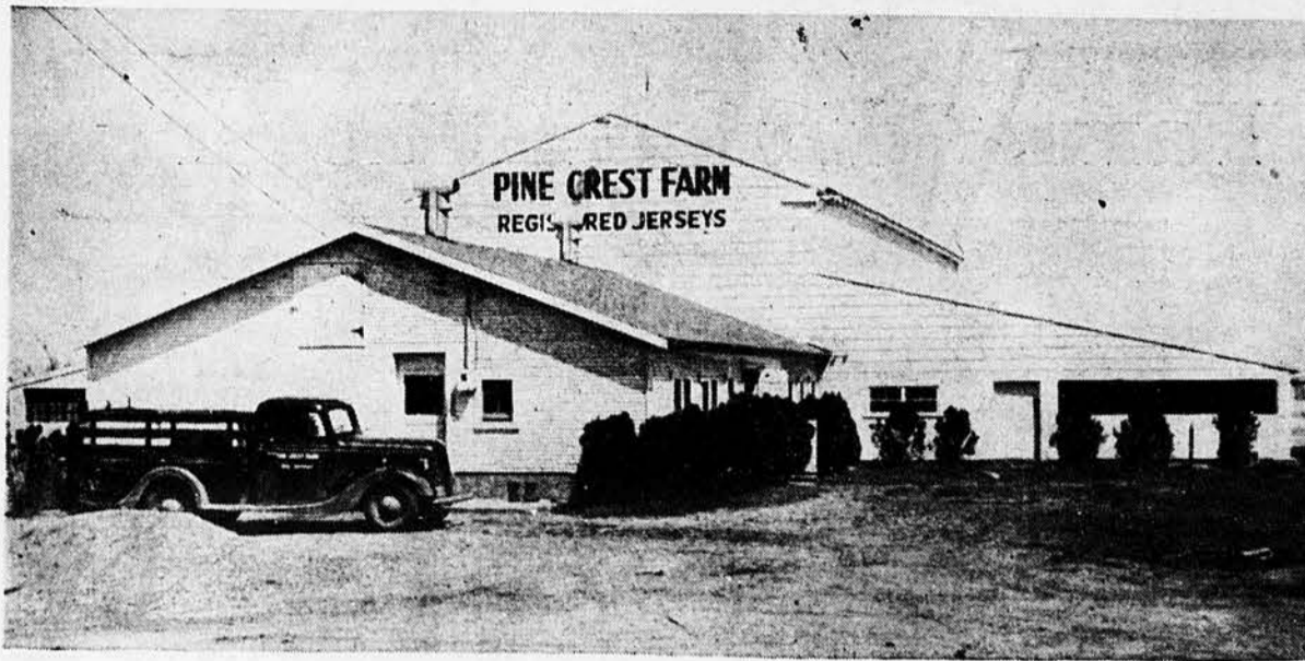
At Left: These attached buildings, on Byler Pine Crest farm, house 12-stanchion, double-row milking parlor in foreground, also hay storage and loafing area in larger buildings in background. There is room for 400 tons of hay in the center of the 84- by 88-foot barn. Loafing sheds on each side are 30 by 84 feet. Dividing gates at entrance to milking parlor bring cows in from one side of loafing barn, shunt them out to other side. Notice maternity ward at far right.
