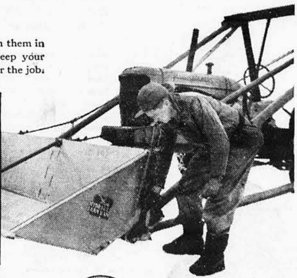
6. V-PLOW. The newest FARMHAND Loader Attachment, and a lifesaver where you've got big plowing jobs to do. Fits on the Loader in a hurry, bucks through the drifts with FARMHAND Hydraulic power to lift and move it over obstructions. More of these specialized FARMHAND attachments are soon coming to speed work, save money for you!
