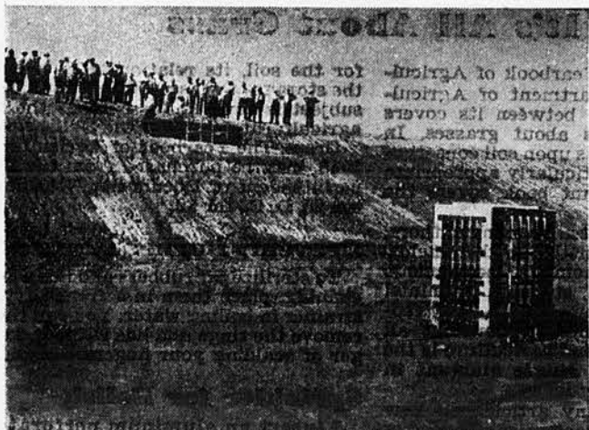
Below: After reaching the temporary reservoir, water is released at a fixed rate thru the concrete outlet, right foreground. An overflow outlet near the top of the dam would take care of extreme flood conditions.
