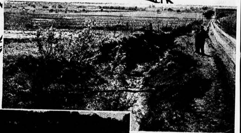
Serious damage to county road in Miami county was caused by discharging terrace runoff into road ditch, a common practice in Eastern Kansas. Damage such as this has cost Miami county up to $600 for one-quarter mile of repair.
