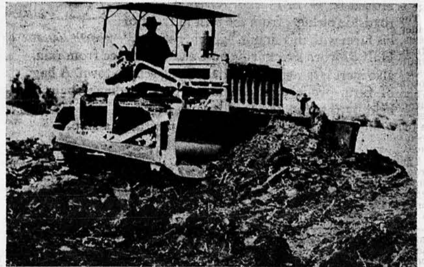
Levelling the top of the terrace with a bulldozer. After levelling, Mr. Northern smooths down the upper and lower slopes by backing his outfit and using the back of the blade. He has built 700 feet of completed terraces in 1½ hours with this outfit.
