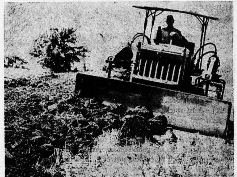
Joe Northern, Miami county contractor, has proved good terraces can be built with a bulldozer. Here he is shown smoothing the down slope.
