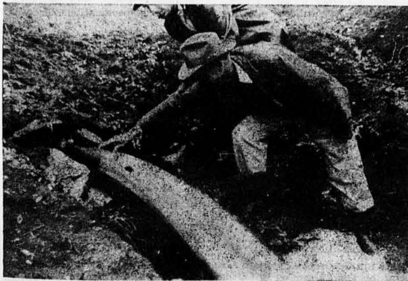
Clarence Ater, former Miami county FHA supervisor, showing amount of water carried by a pond trickle pipe when running at capacity. Installation of a trickle pipe is a highly recommended practice for Eastern Kansas to cut down wave action on dam, and to protect spillway.
