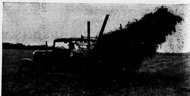
This carrier-type hay buck, built by 2 Nemaha county farmers 3 years ago for $200, will do the work of 3 racks and their crews. The buck will pick up in the windrow, size of load being determined by weight the front end will hold. A load of 1,000 pounds is possible.
