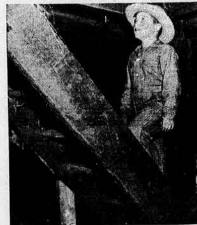
That old ladder to the hay loft has been replaced in the Rohrer barn by this safer stairway. Hugh Rohrer, Clark Creek 4-H Clubber, shows advantages of the stairway.
