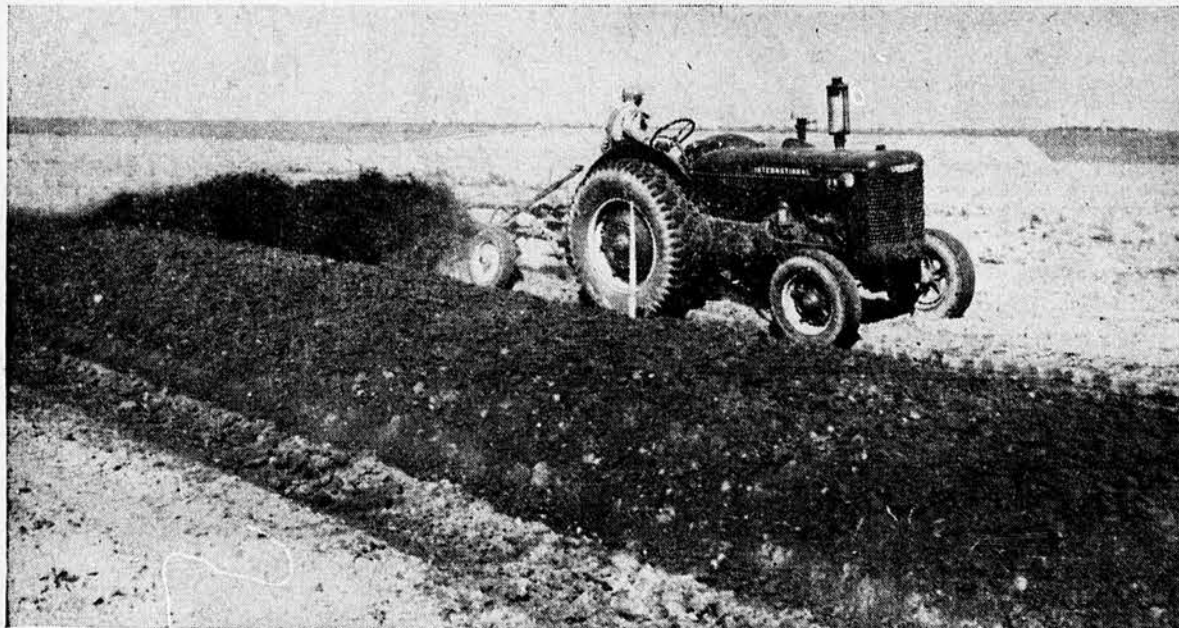
To show visiting farmers how it is done, H. C. Shriner built a terrace at the close of the Trego county tour. He builds terraces for $70 a mile.
