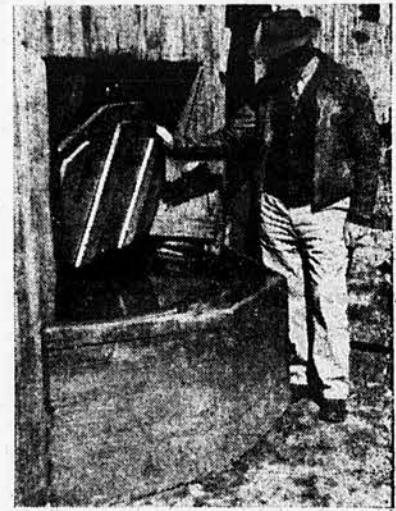
This stock-water tank is built into the barn and is insulated with earth and covered with a lid in winter. Water is pumped to the tank by an electric motor on windmill pump. In front of tank is a concrete floor which prevents a mudhole from forming in the barnlot.
