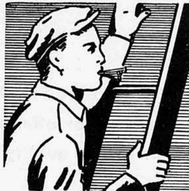
The mouth makes a handy nail pouch; but holding nails in this way is dangerous. One slip, and nails will puncture the holder.
